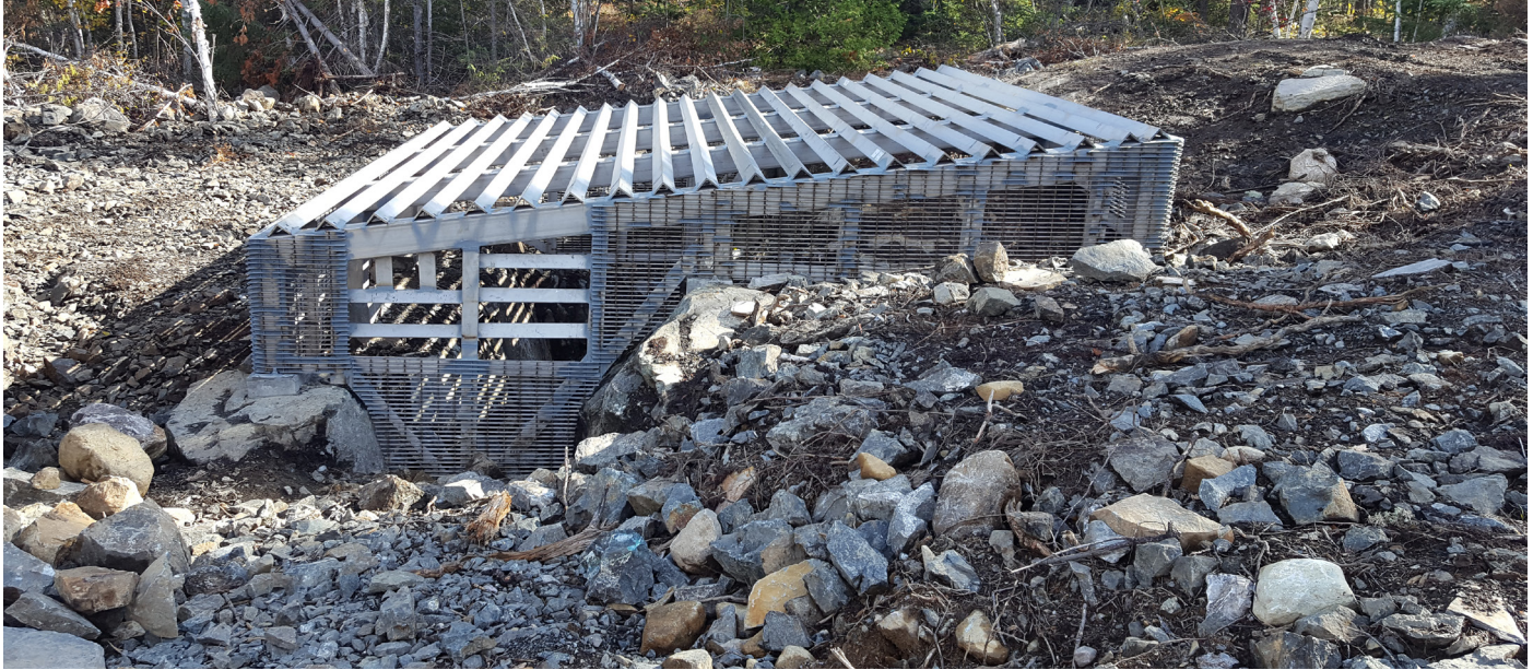
Completed Edison Shaft Cupola – Complete Stainless Steel Construction
