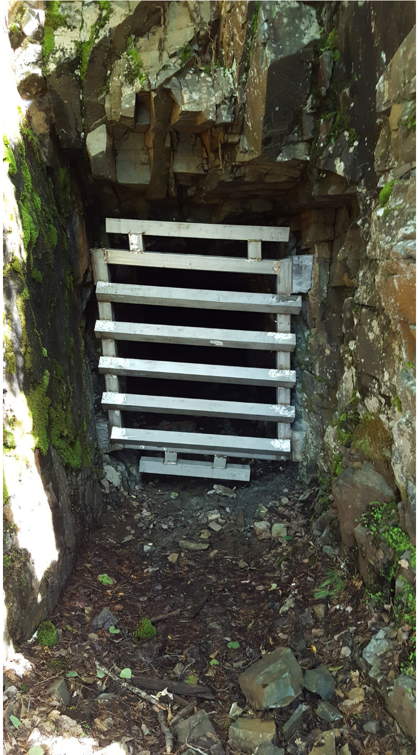
Adit Bat Gate securely anchored into bedrock walls
