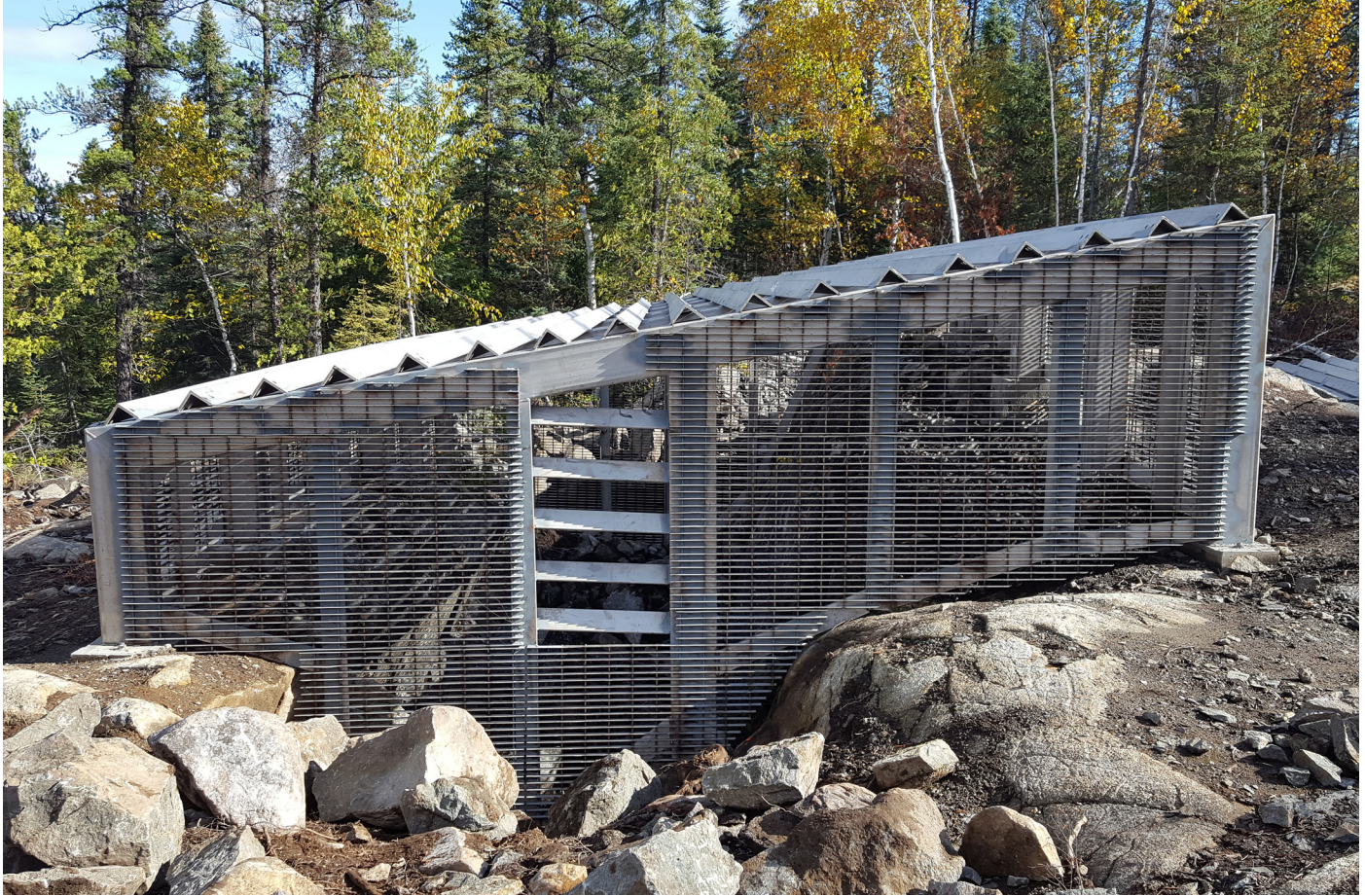
Completed Edison Open Cut Cupola – 146 mm spacing between all steel members
