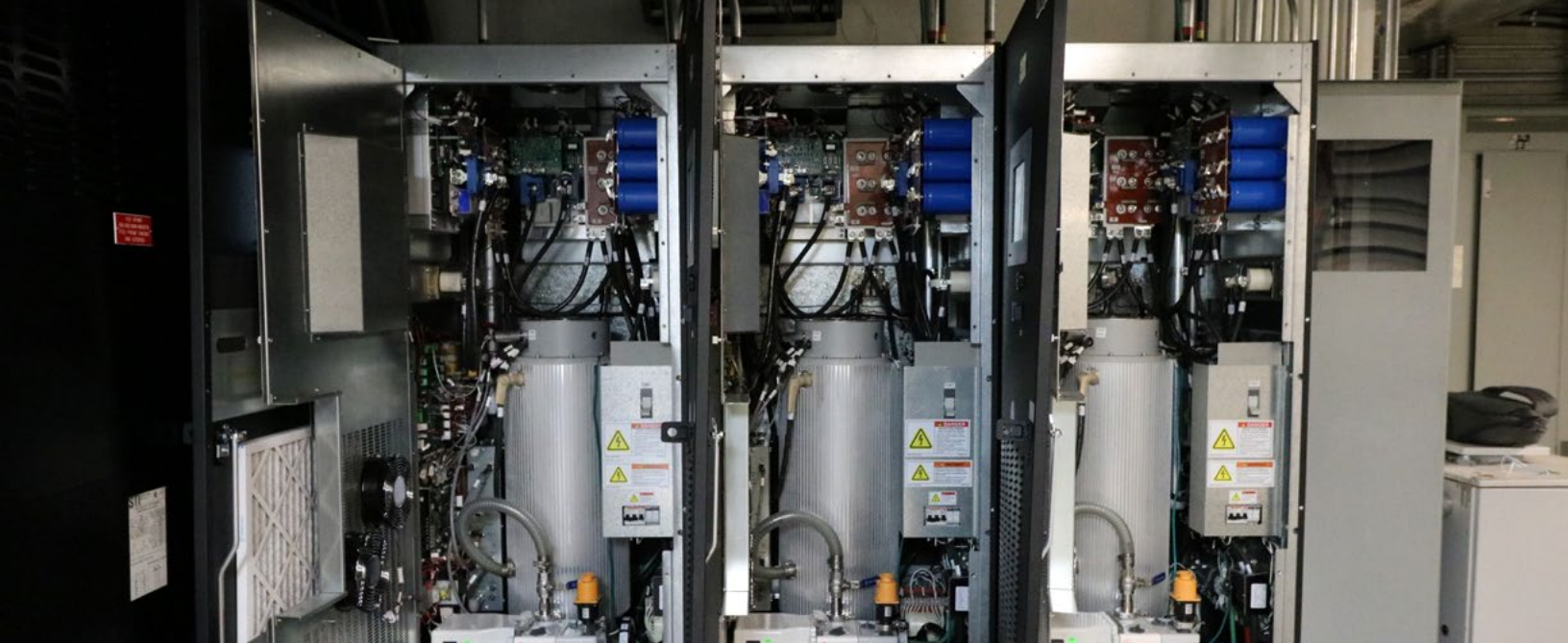
900 kVA Flywheel Energy Storage System
