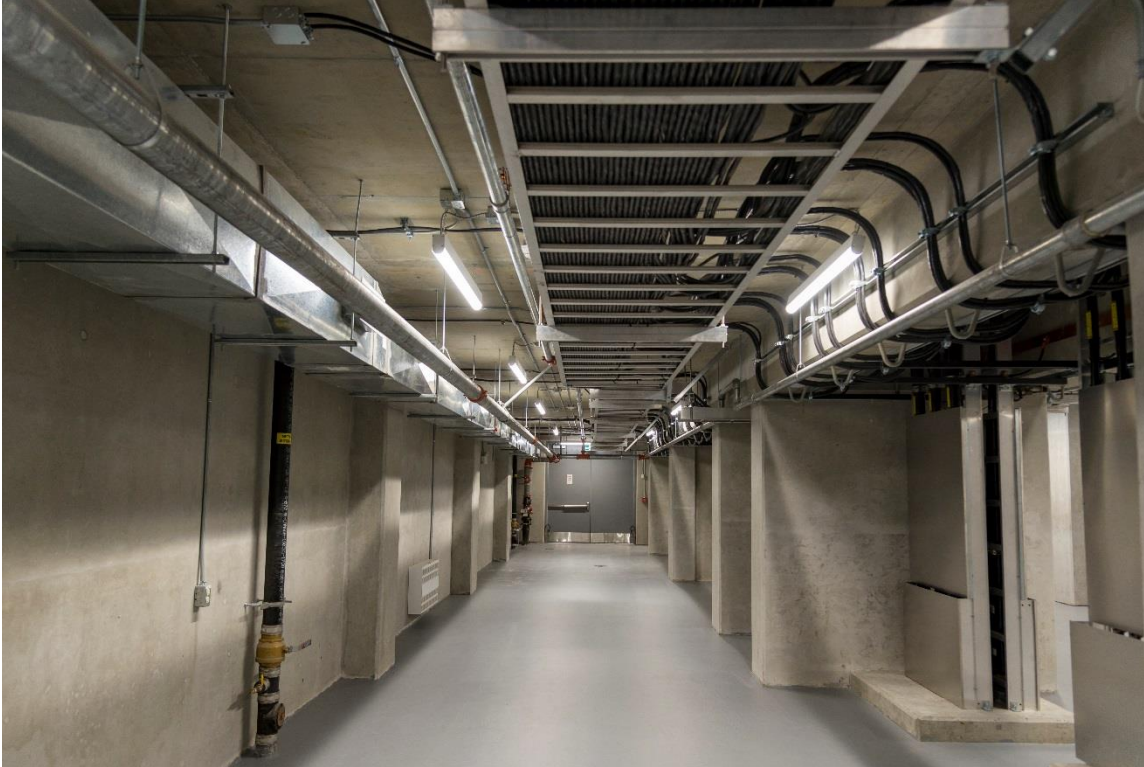
Cable entry to 12kV Feeder Buildings
