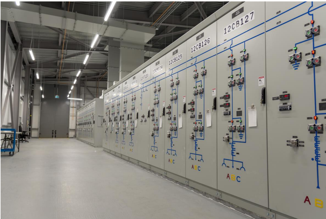
12kV Gas Insulated Switchgear Feeder sections
