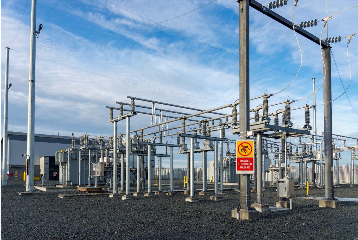
69kV Switchyard and Transformers
