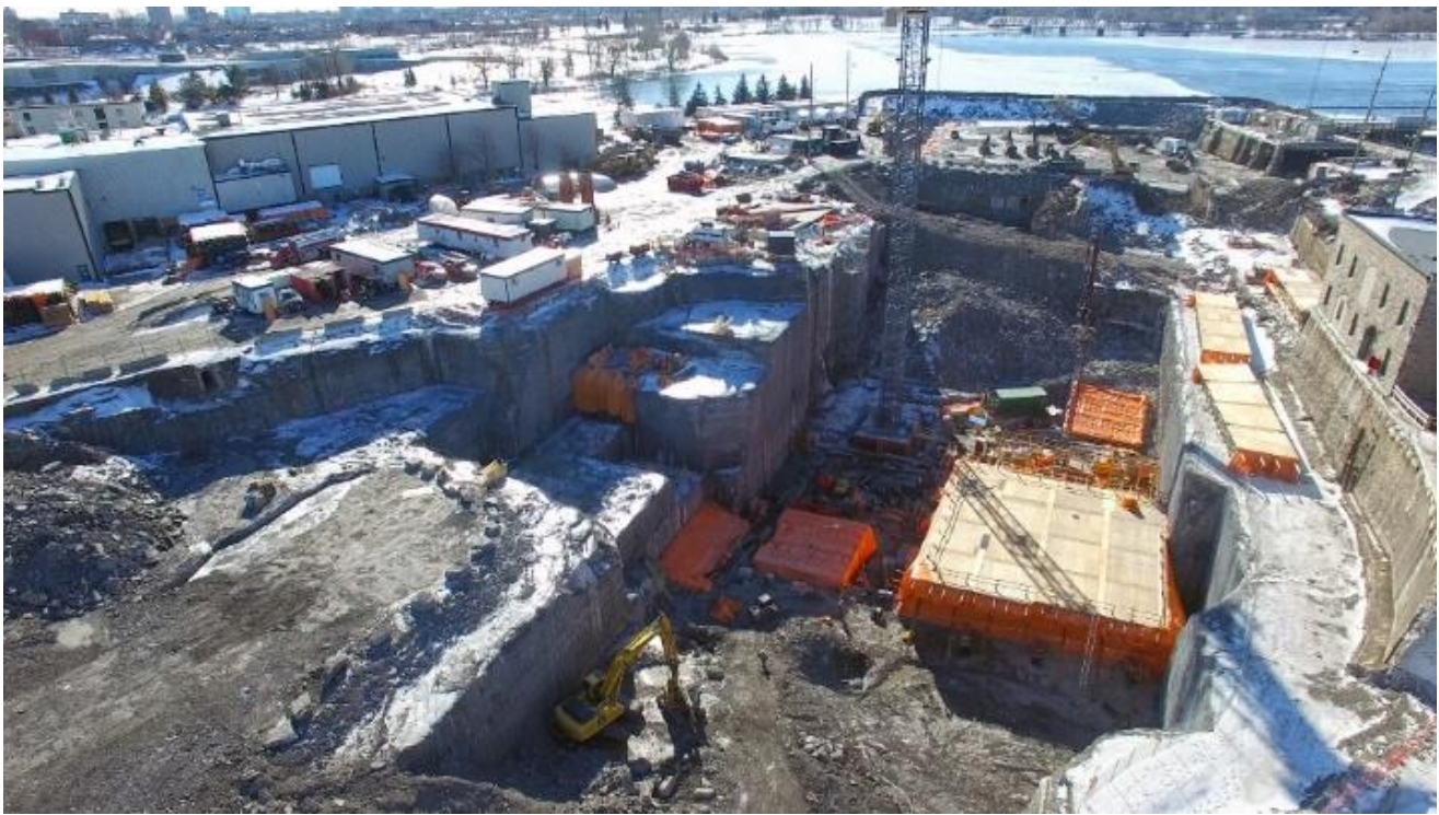
Figure 1: Powerhouse construction starting following excavation
