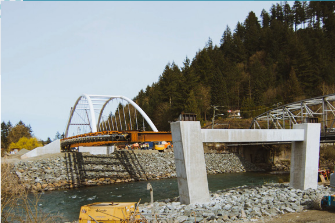
Nose advancing towards the pier on the south bank
