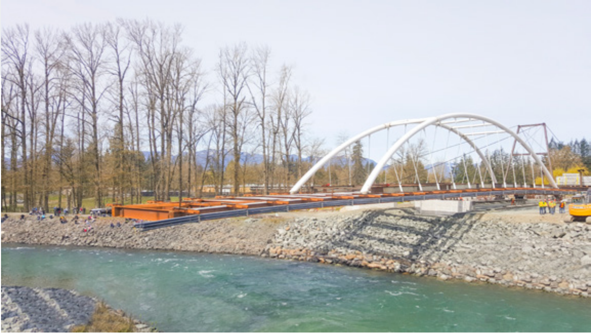
Launching the new bridge across the Vedder River
