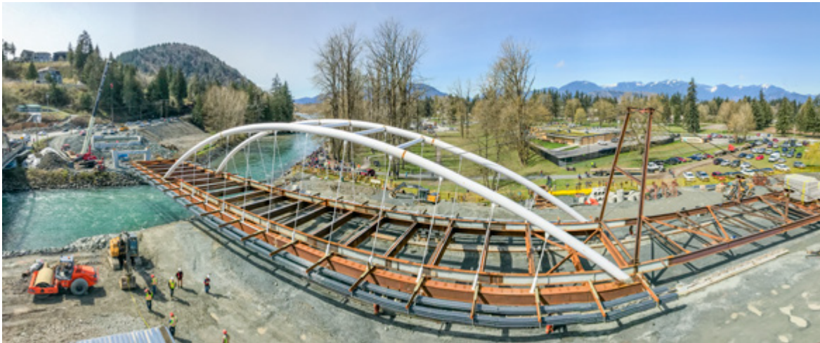
View of the kingpost system and counterweights during launch
