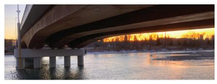
variable depth and a curved vertical profile. With this design, most of the bridge will remain out of water in a 1:100-year event. The structure's shape also improved overall hydraulic capacity of the rivers' cross section, ensuring the structure will not impact water throughput under higher seasonal and flood conditions brought on by climate change.
