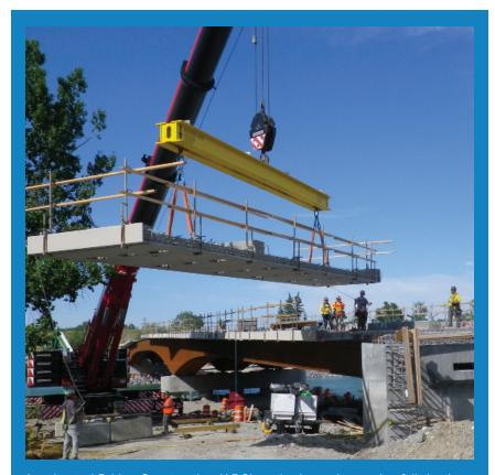
Accelerated Bridge Construction (ABC) methods, such as using full-depth, full-width deck panels combined with Ultra High-Performance Concrete, are increasingly common tools for bridge designers. There are several benefits from using precast ABC techniques, including a higher level of quality control compared to traditional cast-in-place elements, less onsite formwork, shorter construction timelines, and lower risks corresponding to work over water or live heavy traffic.
