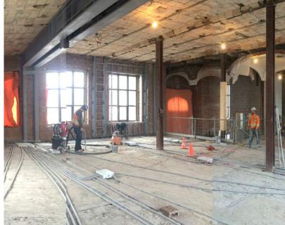
The masonry restoration was an important component of the renovation, as the walls act as both the building envelope and the lateral load resisting system.
