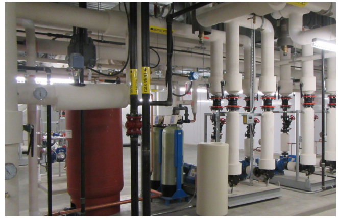
Mechanical System Circulation Pumps
