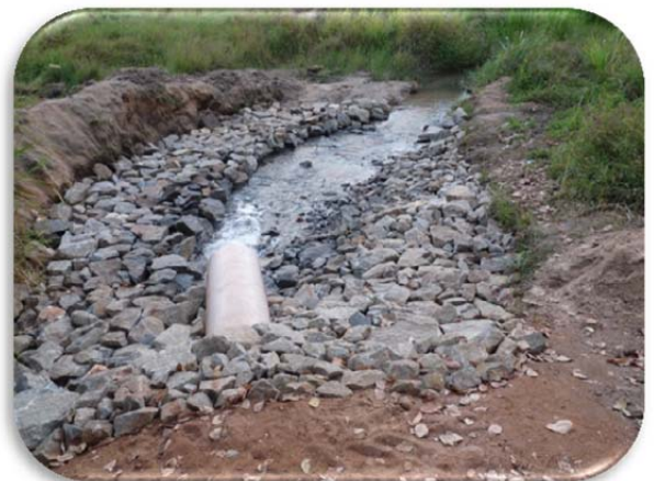
Erosion protection at the outfall from the solids management lagoons at the Nampula water treatment plant
