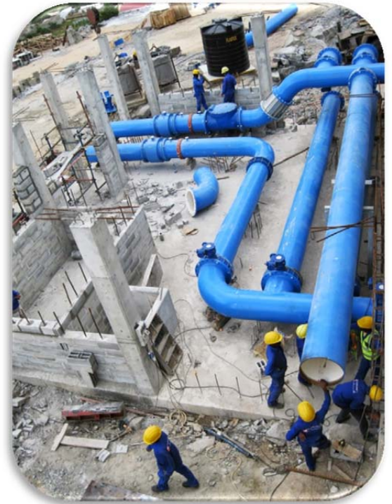
Workers install pipes at the new 5 ML reservoir, designated as “EB5” in Nampula
