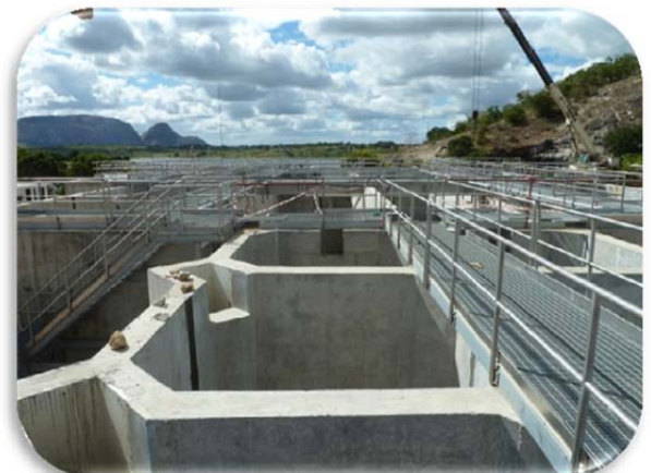
Hydraulic flocculators designed by Burnside based on Canadian technology and implemented in Nampula, Mozambique
