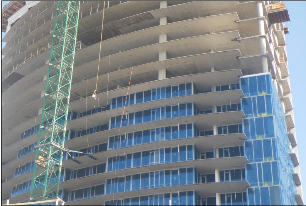
Photo 2: From BETB Guide: example of common residential high-rise with extended concrete floor slabs around perimeter and building envelope of mainly floor to ceiling window-wall.
