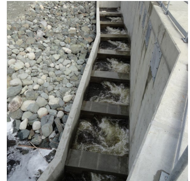
Vertical slotted fish ladder, operation of downstream section
