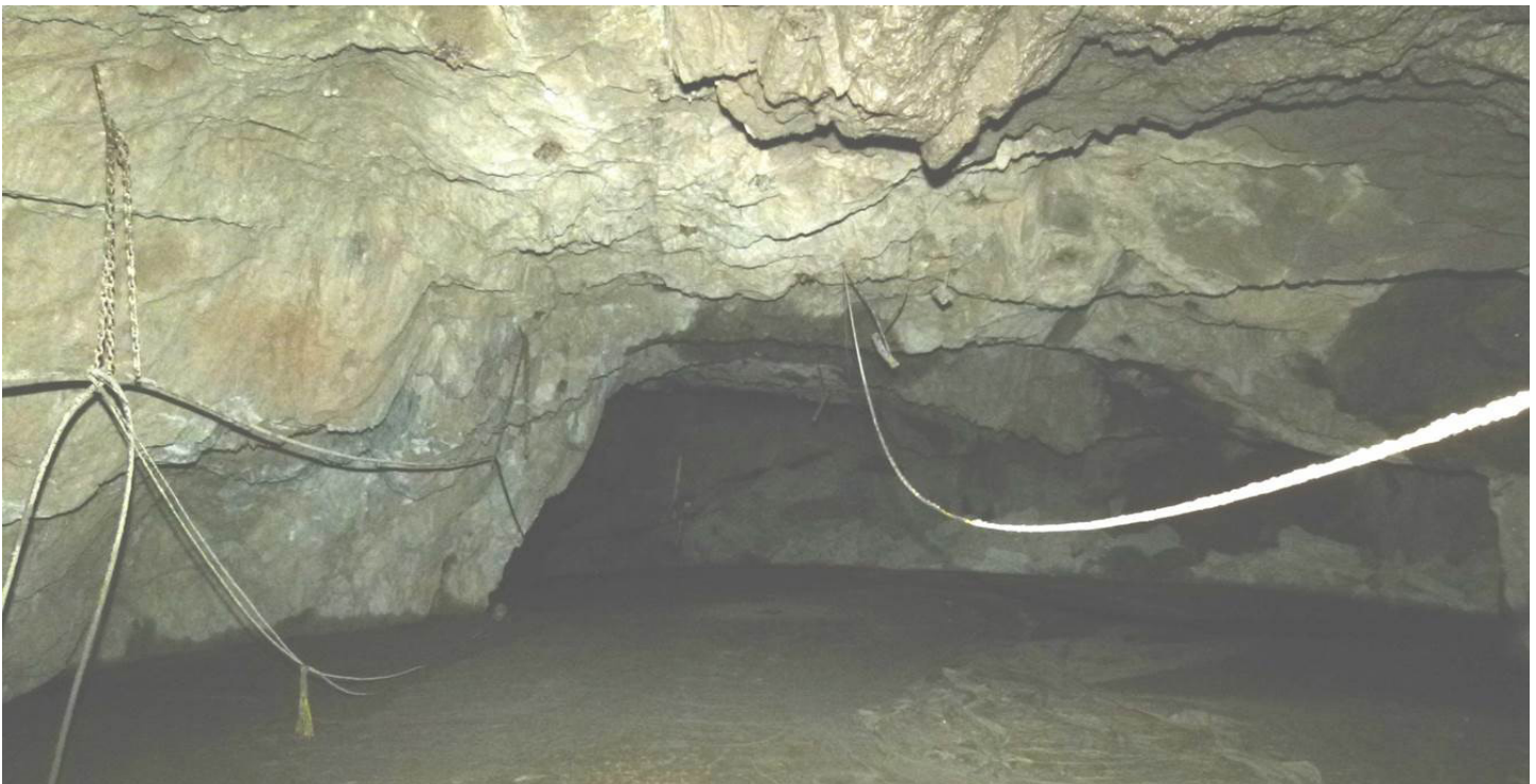
Photo 12 - Partially Backfilled Stope Void Under Baker Creek
