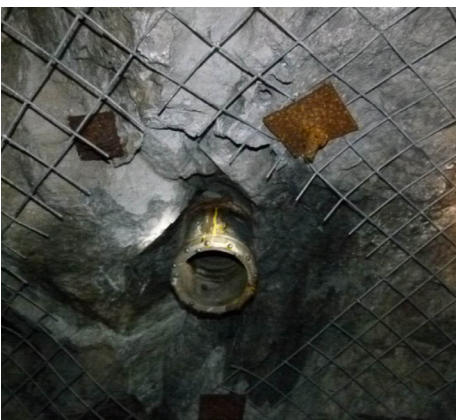
Photo 7 - Underground Breakthrough of 50 m Long Borehole With Steel Casing From Surface
