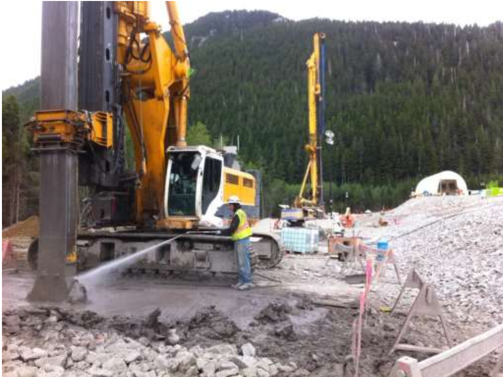
Image 9: BG36 cutter head exiting completed panel
