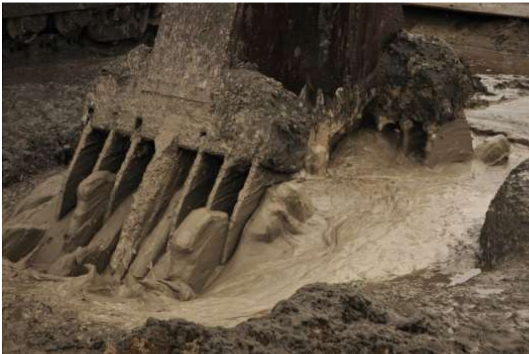
Image 2: Cement slurry mixing with in-situ materials
