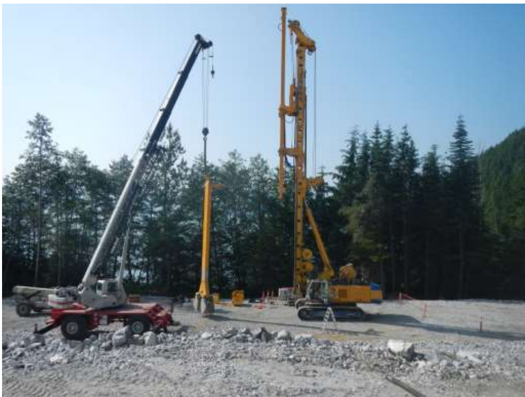
Image 10: Connecting BCM10 Cutter head to BG36 drill rig at start of project
