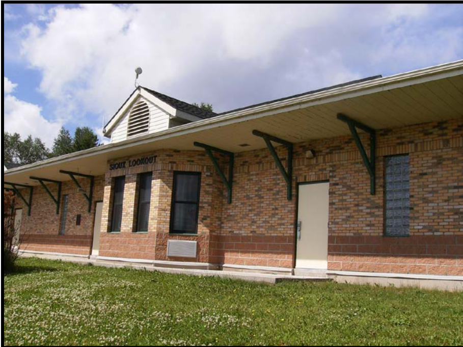
1. Sioux Lookout Water Treatment Plant
