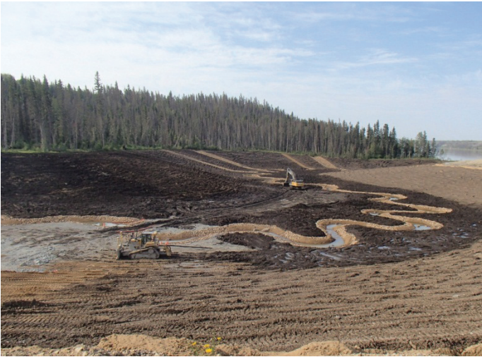
Photo 7: View of meandering outlet channel during its construction, Photo by Golder.
