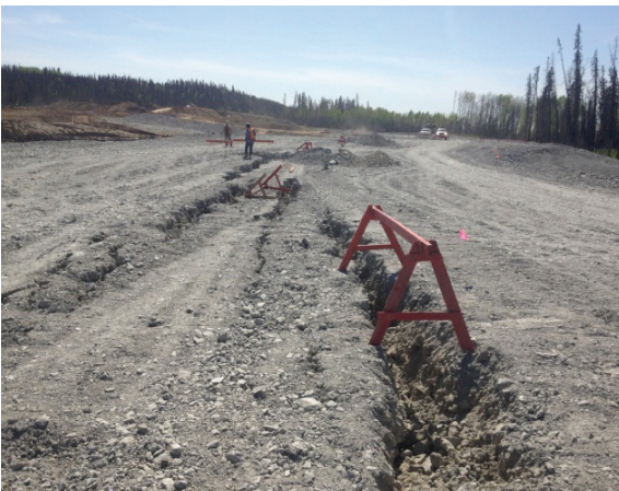
Photo 3: Cracks along the earthfill structure due to settling
