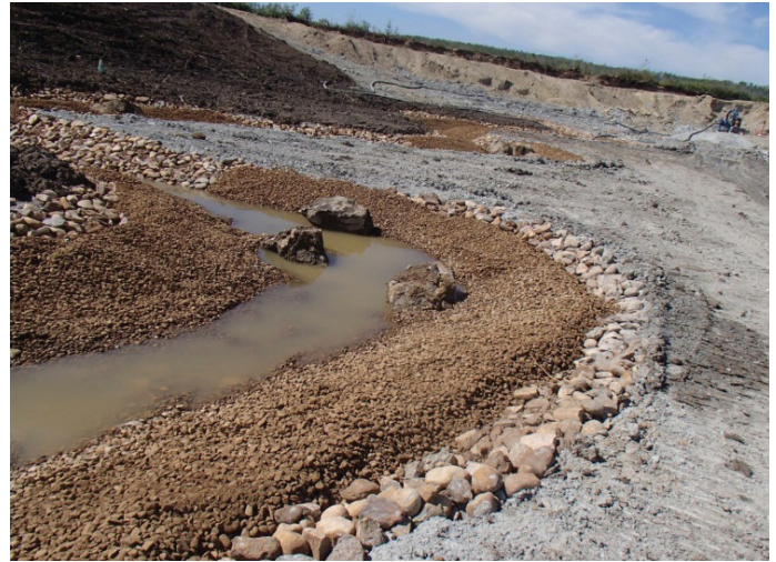
Photo 8: Close up of outlet channel showing fish habitat materials, Photo by Golder.
