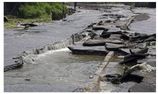
Photo 3 - Road washout after the flood.
