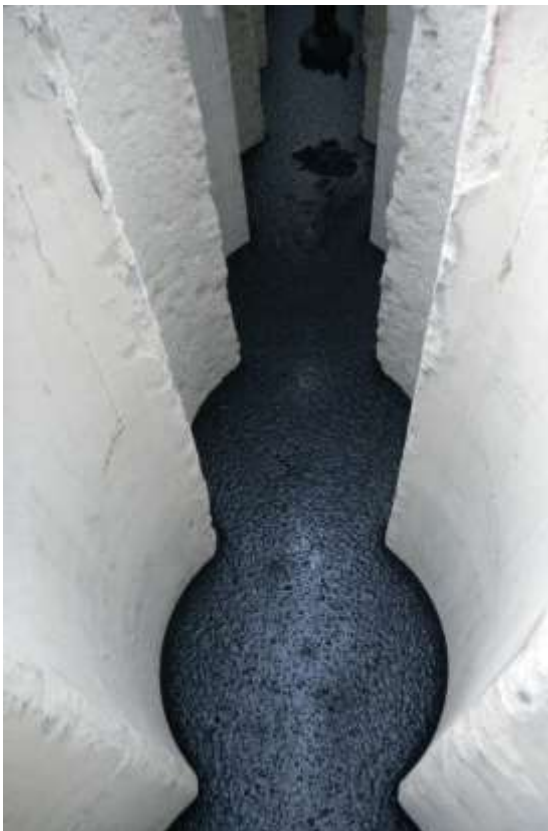
Image 8: Completed Tie-in slot showing mastic asphalt membrane
