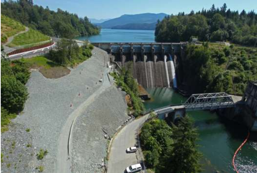
Image 1: Location of right abutment at Ruskin
