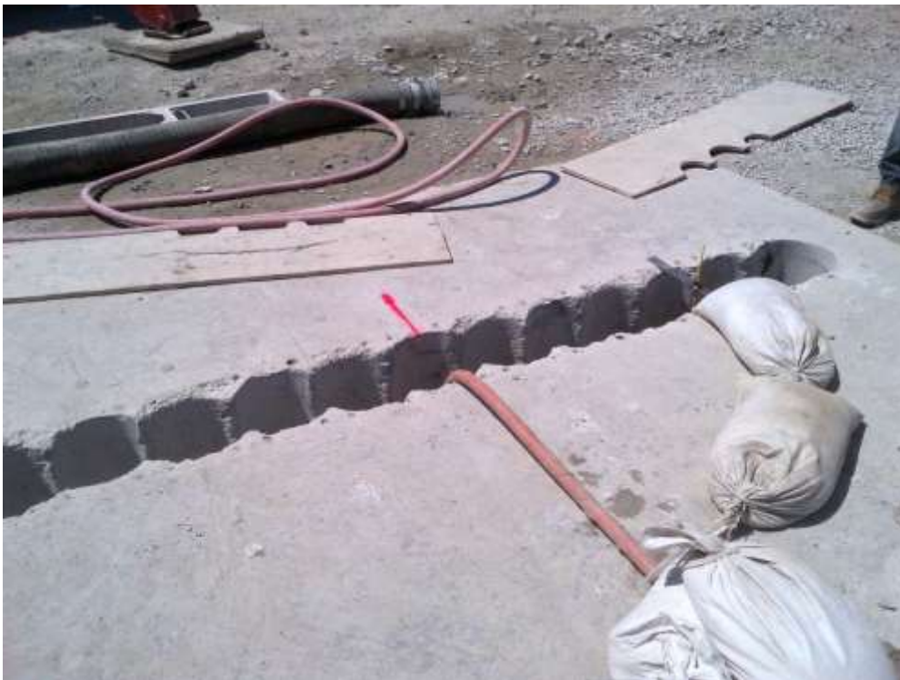
Image 4: Close up of completed overlapping drill holes
