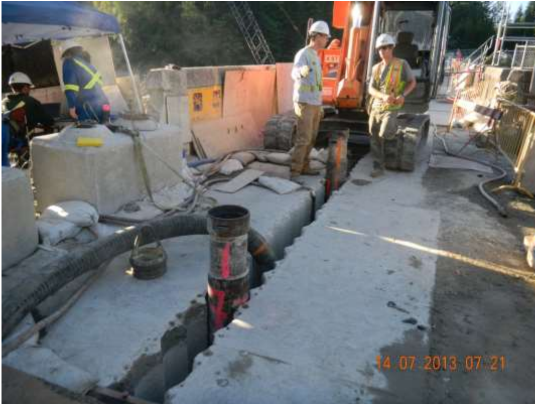
Image 5: Final preparation for mastic asphalt installation
