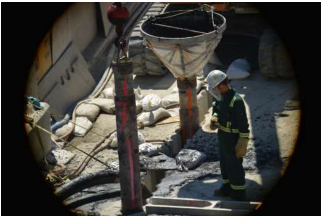
Image 6: Delivery pipes and hopper during mastic asphalt installation
