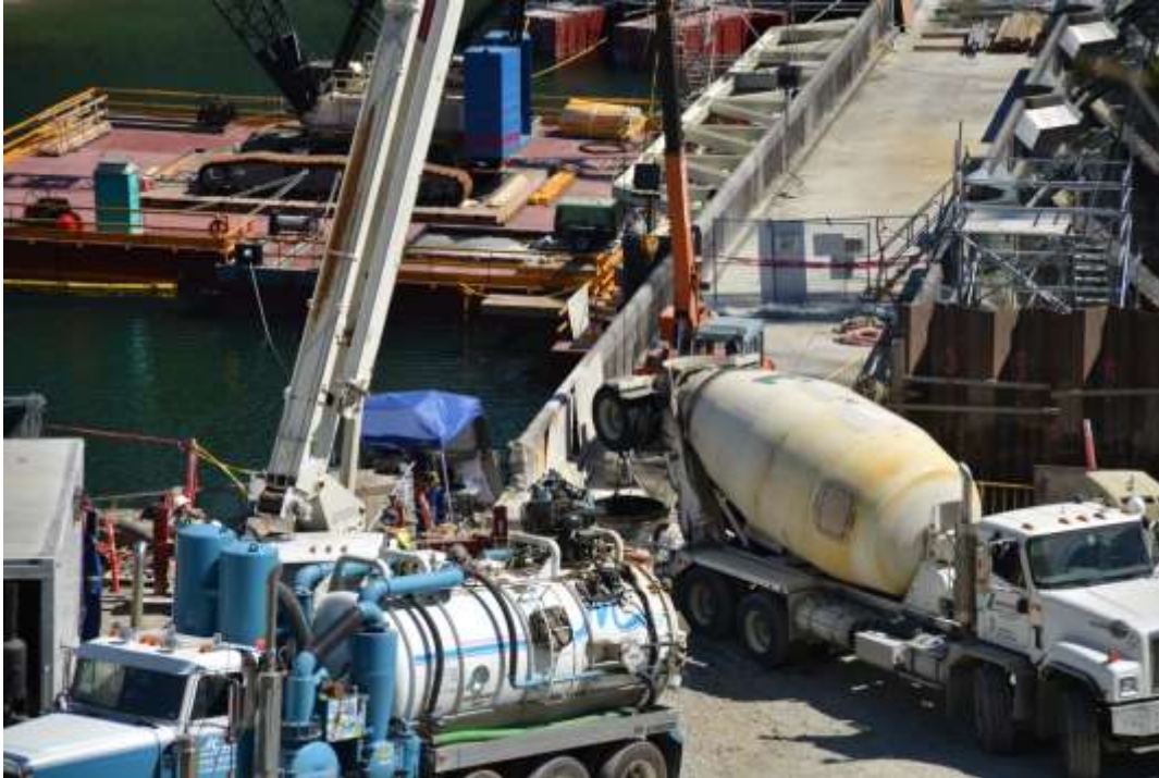
Image 7: Constrained work area showing ready-mix truck delivering mastic asphalt
