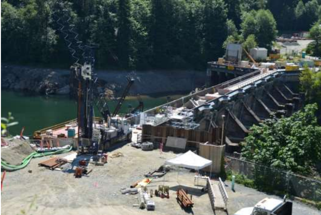
Image 3: Drill rig positioned over tie-in slot during secondary ream out
