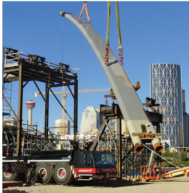
Erection of arch segments
