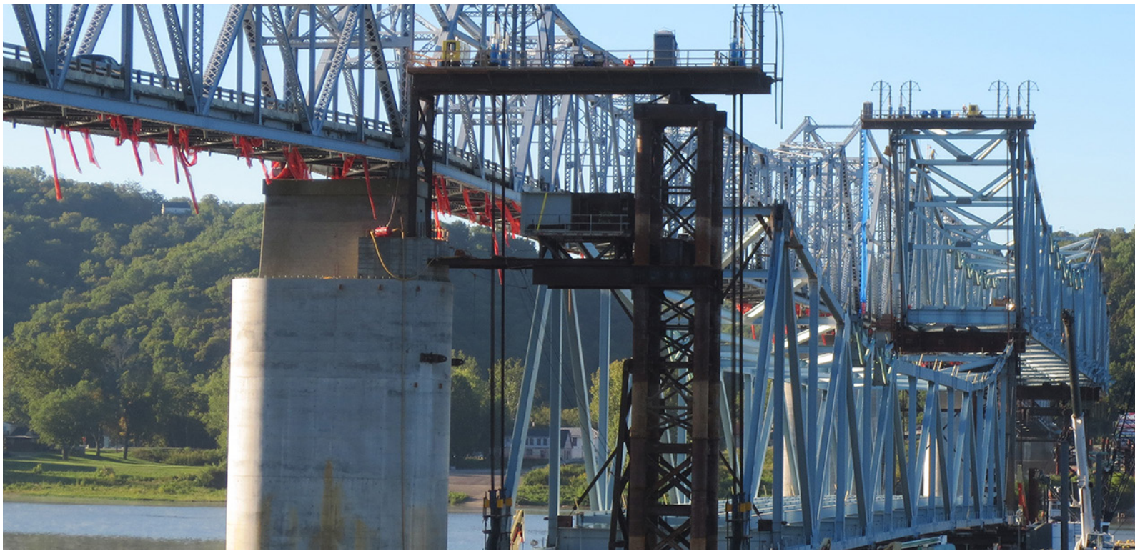
THE NEW TRUSSES BEING FLATED IN NEXT TO THE EXISTING MILTON- MADISON BRIDGE
