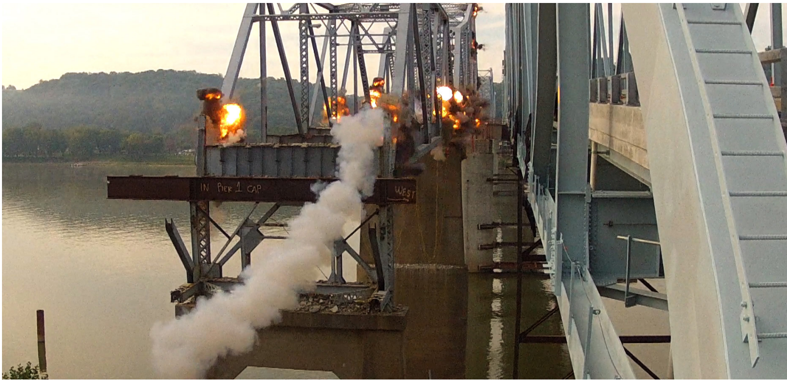
DEMOLITION OF THE OLD MILTON- MADISON BRIDGE NEXT TO THE NEW STRUCTURE
