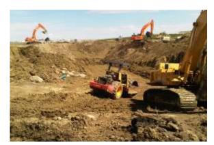
concrete was re-used on site instead of importing crushed granular materials for maintaining roadways and construction haul routes.
