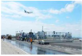
performance for aircraft take-off and landing. Within the overall 400,000 cubic metres concrete paving, over 300,000 cubic metres was completed during a five month period; and 55,000 cubic metres was completed in 3 weeks during the summer 2013 to achieve the project schedule. On our record paving day, over 5,000 cubic metres was placed during a 24 hour period – more production than any other concrete paving project in Canada.
