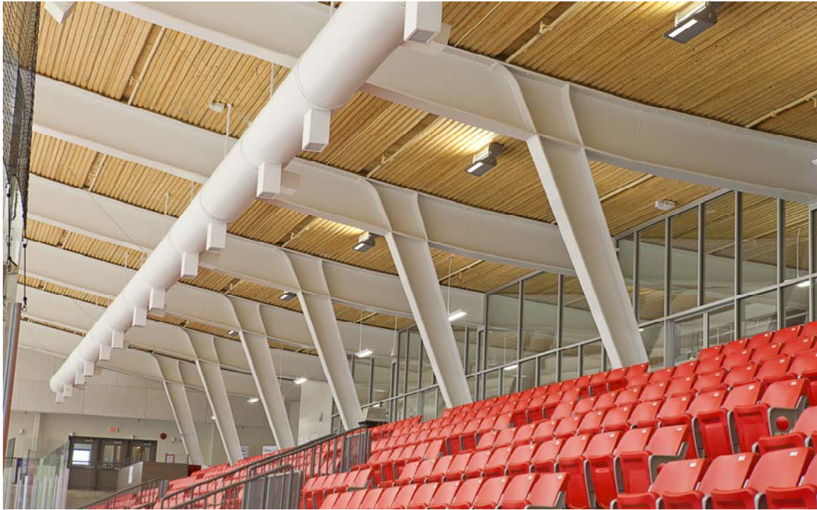
Photo 6: Sloped/sculpted steel columns
