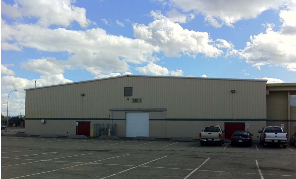
Photo 1: Existing Kin 1 Arena prior to demolition
