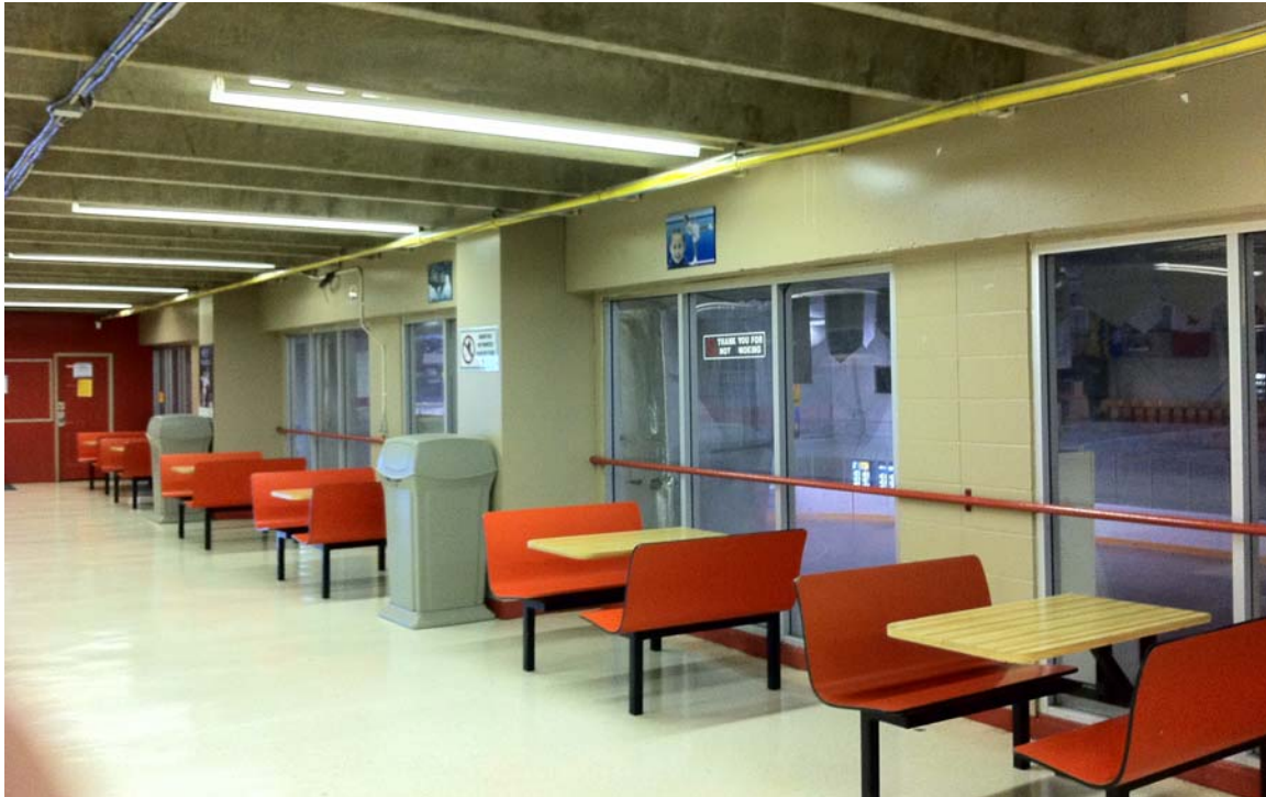
Photo 2: Existing spectator lounge prior to demolition
