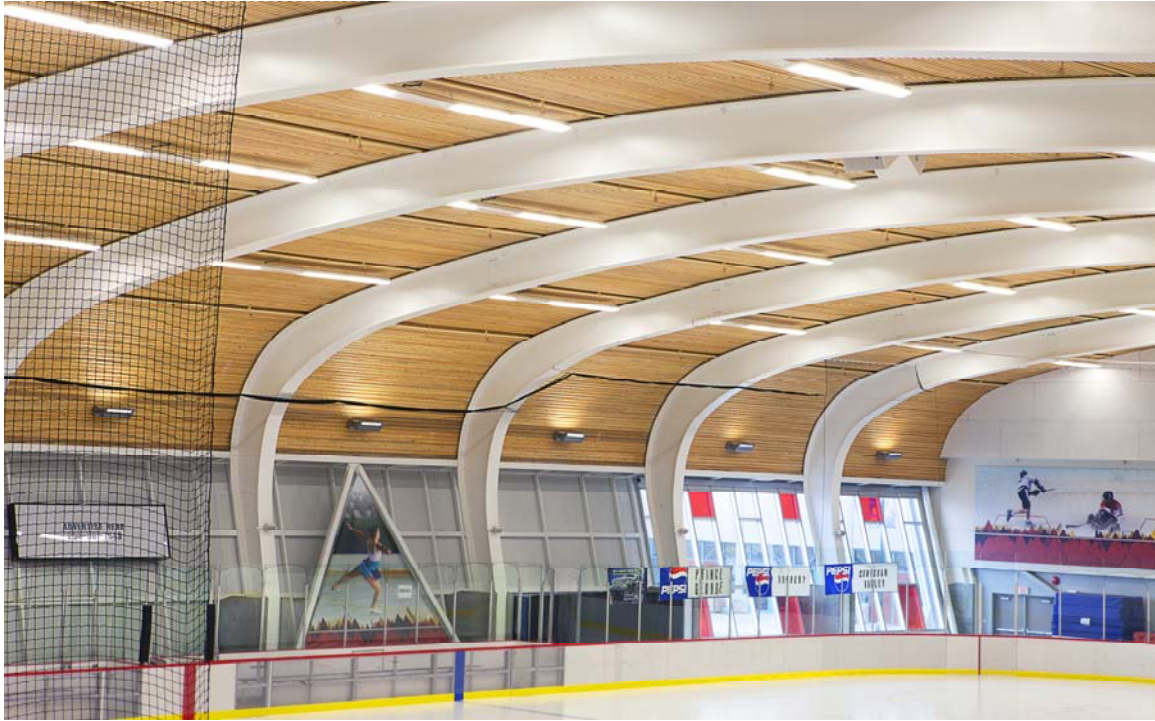
Photo 5: Curved steel beam and solid wood roof
