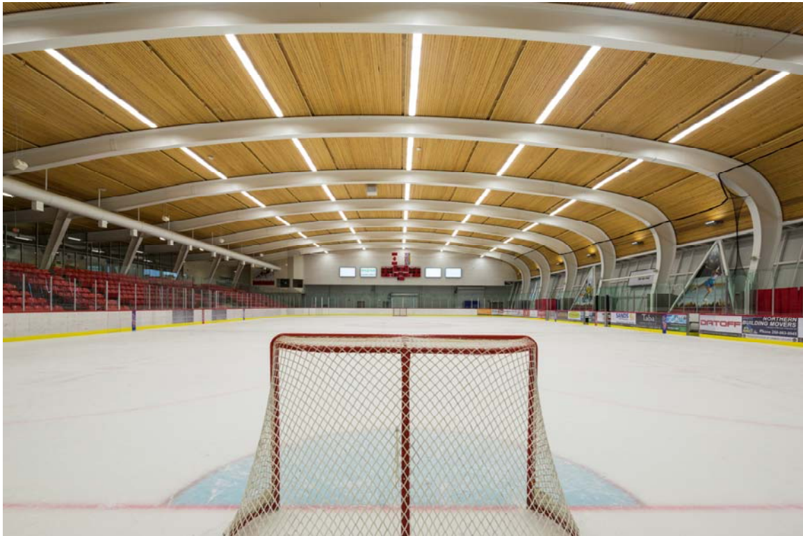
Photo 4: Kin 1 reconstruction complete
