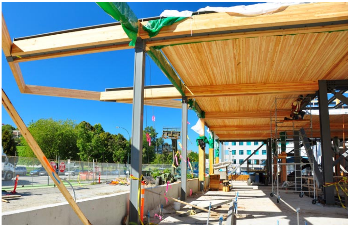
Photo 8: Cantilevered floor framing over bike path.
