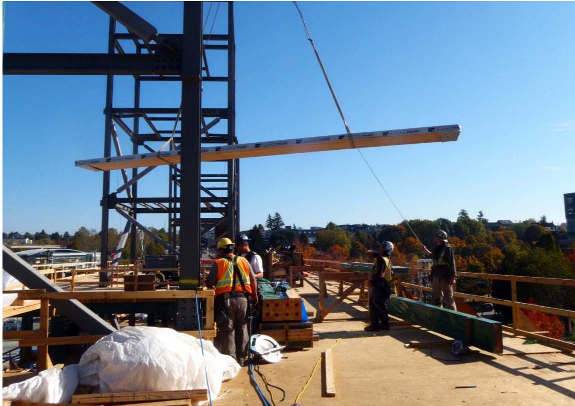
Photo 6: Solid wood panel construction.
