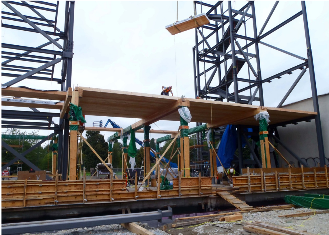
Photo 7: Mass timber floor framing in progress.
