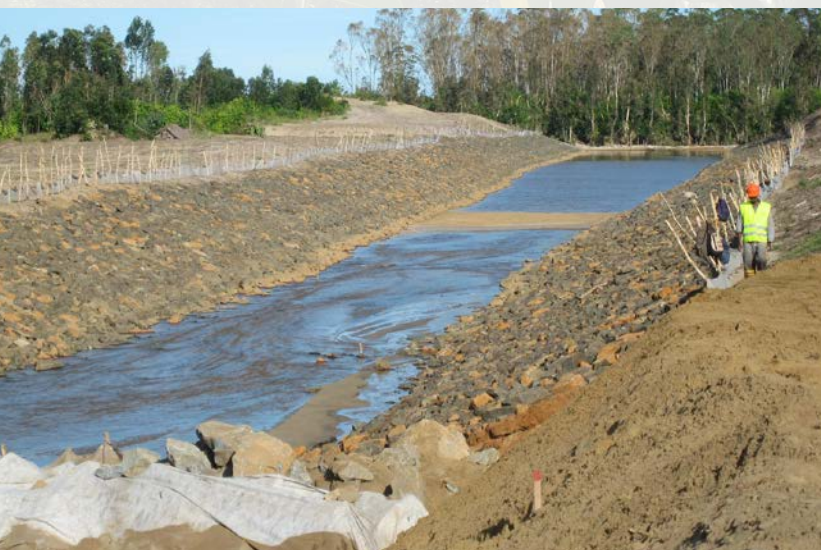
Site dewatering and erosion control
