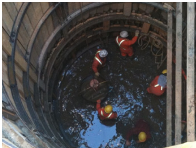
Wet and sticky ground conditions encountered during portal construction
