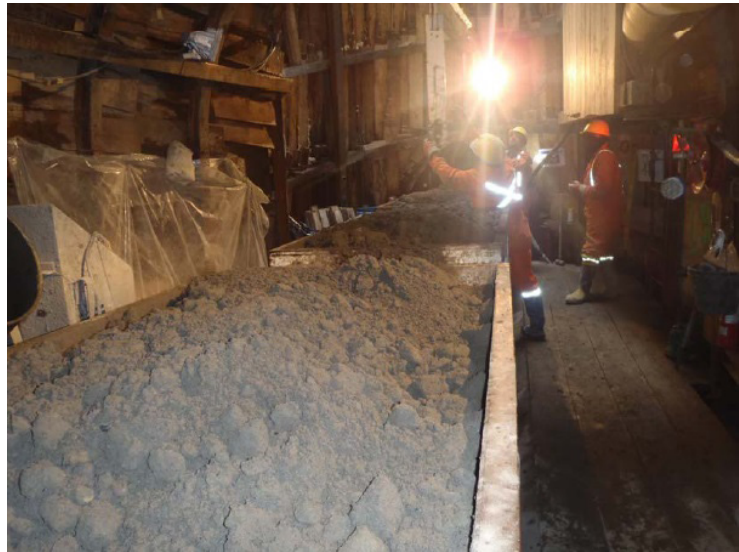
Removing debris from the portal storm tunnel excavation
