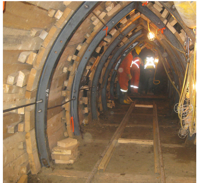
Hand tunnelling in the double barrel tunnel
