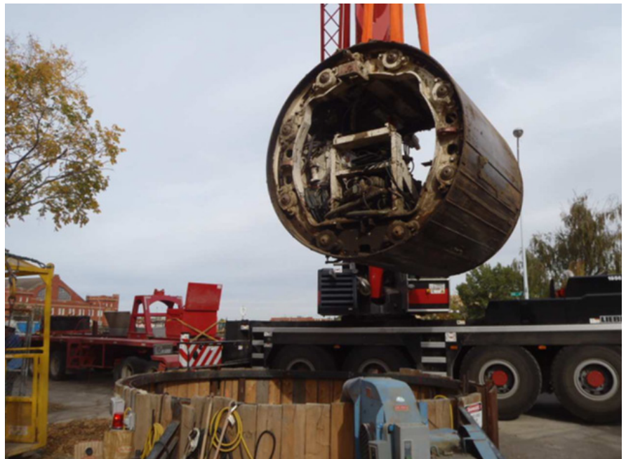
Removing TBM from portal tunnel
