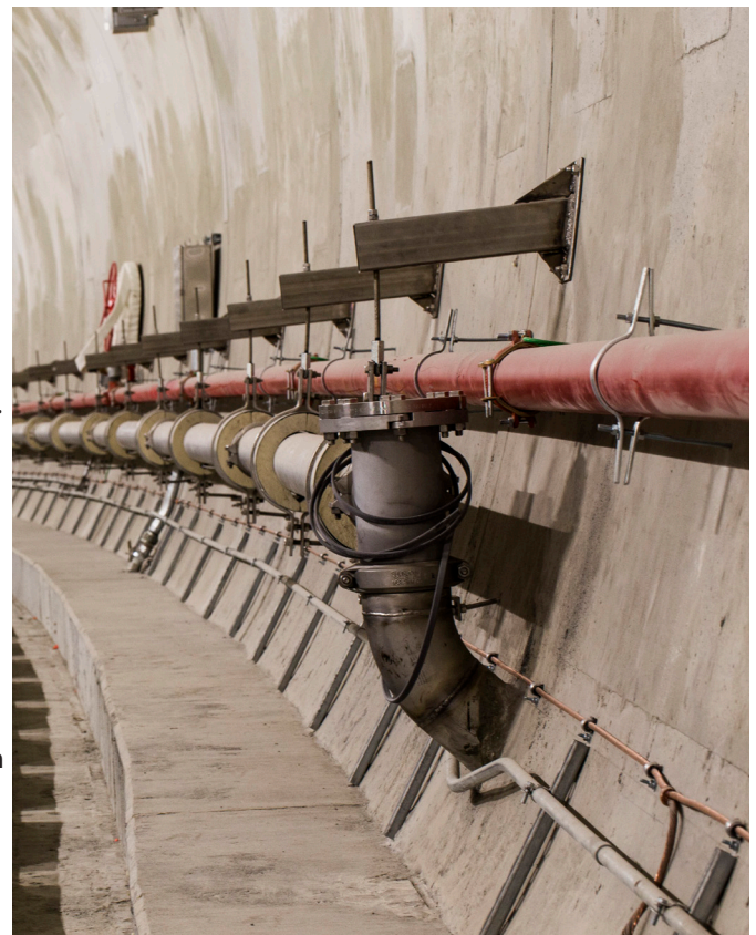
Drainage for the North LRT tunnel built as part of the double barrel relocation
