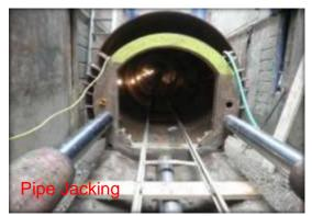
Several types of trenchless technology, including pipe jacking, hand mining, and micro-tunneling, were used on this project. Hand mining and pipe jacking was successfully implemented in most areas with varying ground conditions which allowed the miners to have full access to the
