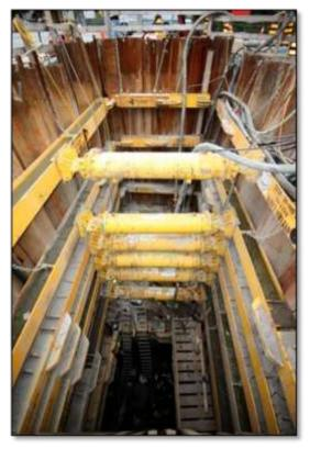
Excavating deep shafts, some within two lanes of traffic, was a notable challenge. Complicating matters was the previously disturbed nature of much of the tunneled silts and sands from previous construction, both below and above the tunneling alignment.
