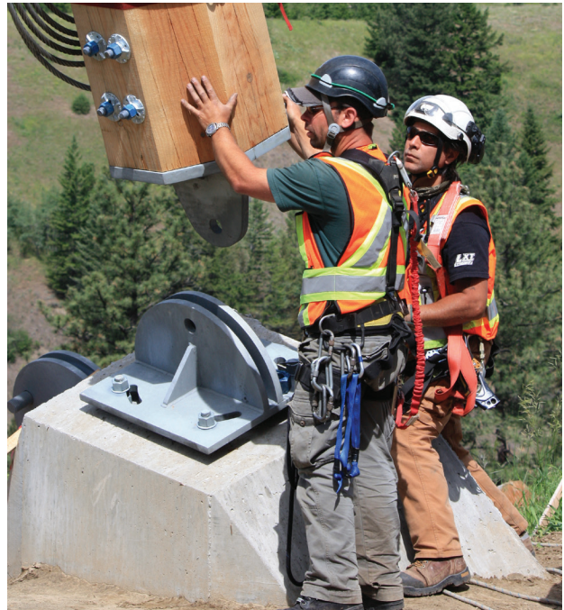
The Primal Swing was supported on micro-piles to reduce ground disturbance and the risk of site erosion
