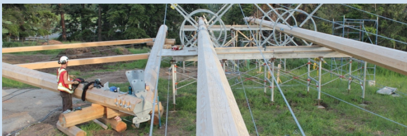
Assembling the steel trussing around the 8-sided timber
