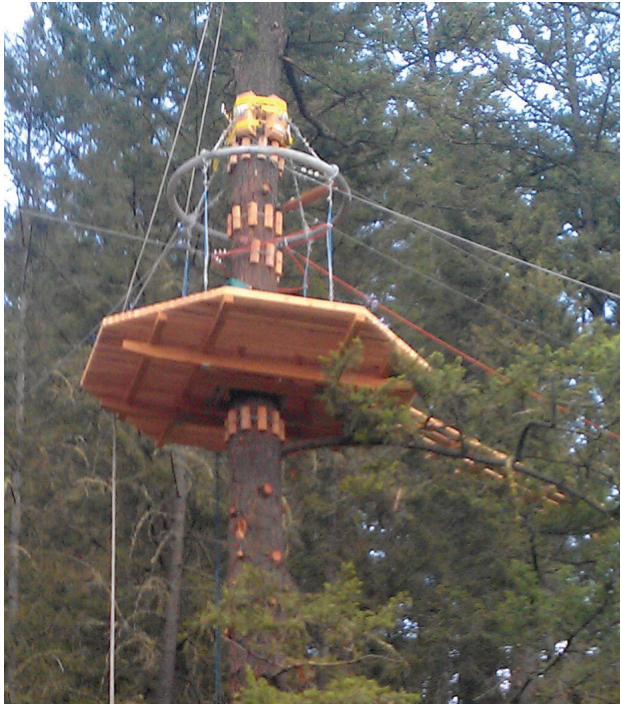
The DragonFLY zipline platform connections were designed to clamp on using friction rather than mechanical fasteners, limiting damage to the trees
