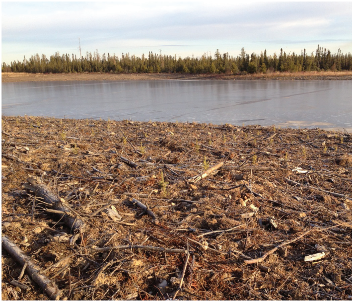
Photo 3: Woody debris spread on the reclaimed slopes to enhance biodiversity and revegetation success
