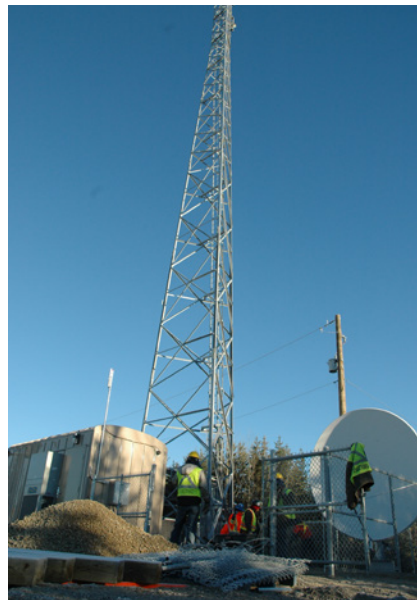
Construction of a 150 ft. antenna and a 12 ft. dish
