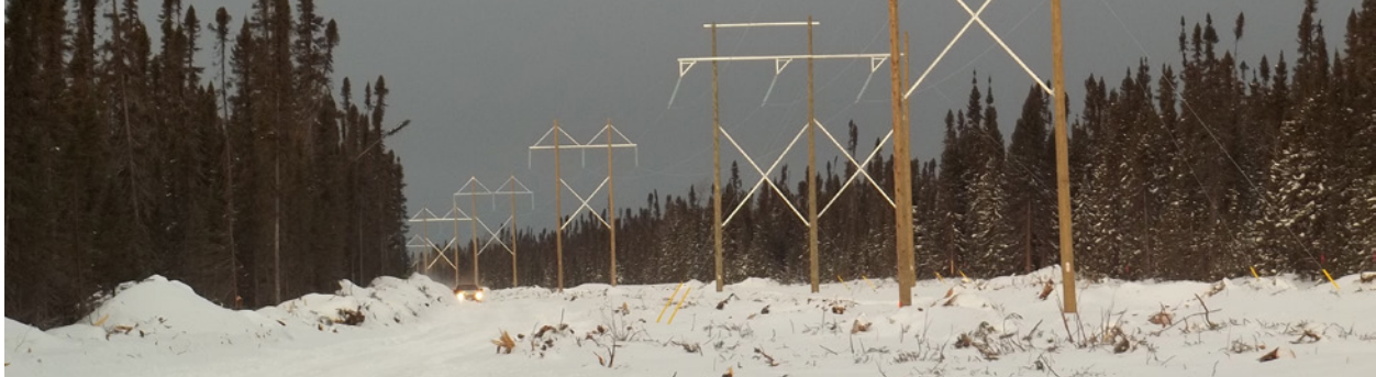
Line built during winter due to important muskox and sensitive wetland features.
