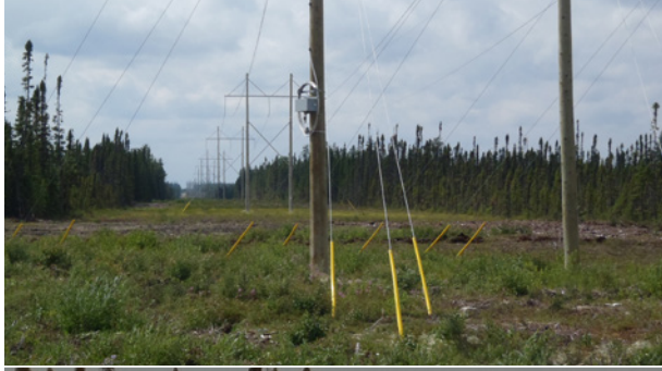
The mine is fed through a 230 kV, 180 km-long power transmission line.
