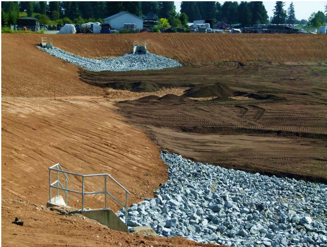
Photo 3 – The Infiltration Gallery under Construction – View 2
