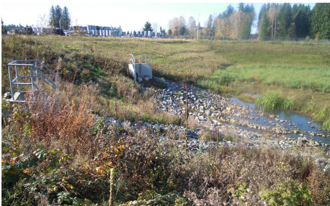
Photo 5 – Inlet Structure with Energy Dissipating Rock Channel
