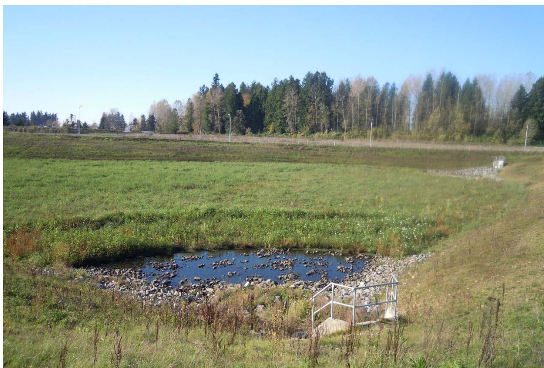
Photo 6 – Sediment Pond and Initial Infiltration Zone (Typical at each inlet)
