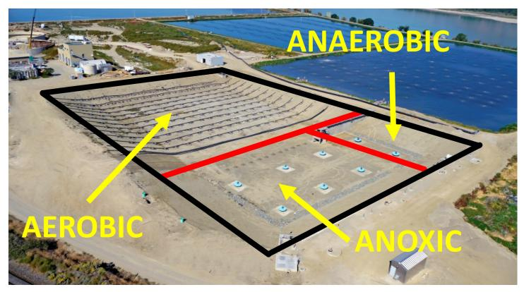
Figure 3: Modified and reduced size Cell with mixing and aeration equipment in place, prior to installing the baffles to partition the lagoon into the three separate environmental cells required for biological nutrient removal.
