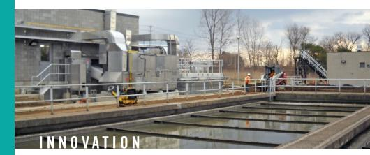
The Vauxhall PCP is one of the first Ontario municipal wastewater treatment plants to have implemented a wet weather strategy that involves flow diversion, chemically enhanced primary treatment (CEPT) and chemically enhanced secondary clarification processes. The \$5.6M plant upgraded pulled together technologies already in use by the industry and reimagined them for this application in such a way that minimal new equipment was required that provided the City of London with cost savings.
