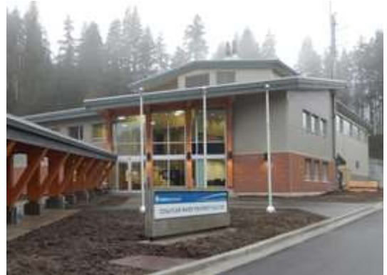
Constructed on a compact site in an environmentally sensitive watershed, this innovative UV Disinfection Facility services one third of MV's water needs.
