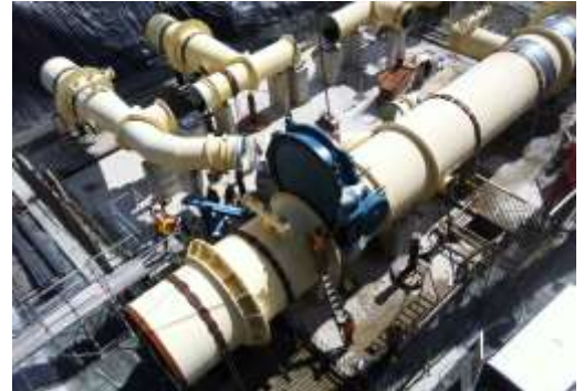
The 3m-diameter (120") butterfly valve which was installed in the intake pipe is the largest valve in the MV system.
