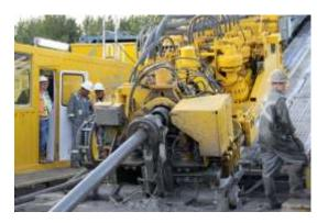
To confirm the appropriateness of horizontal directional drilling, the project team performed a detailed field investigation along the preliminary drill path. Based on borehole data from the field investigation, the team selected an alignment for which
