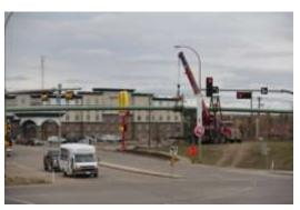
Working closely with the contractor and municipality, the team helped to coordinate the complex roadside erection of steel A-frame structures that would provide support for the pipe string.
