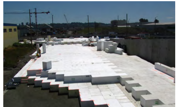
The Project required 280,000 m 3 of EPS, believed to be the largest volume of EPS used on a single North American project.
