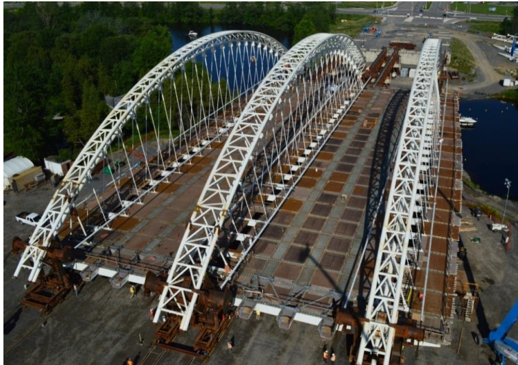
Figure 7. Aerial view of bridge during launching across the Rideau River.
