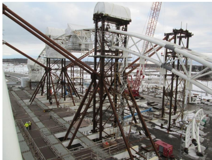
Figure 4. Shoring towers supporting centre arch during construction.
