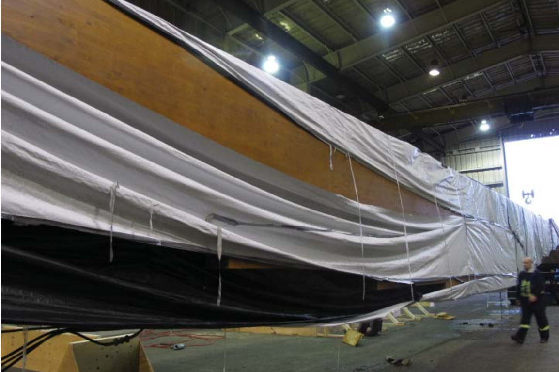
Figure 3&4: Transportation of prefabricated bridge sections. Photo Credit: StructureCraft Builders
