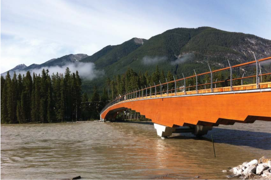
Figure 1: Side view of completed bridge. Photo Credit: StructureCraft Builders
