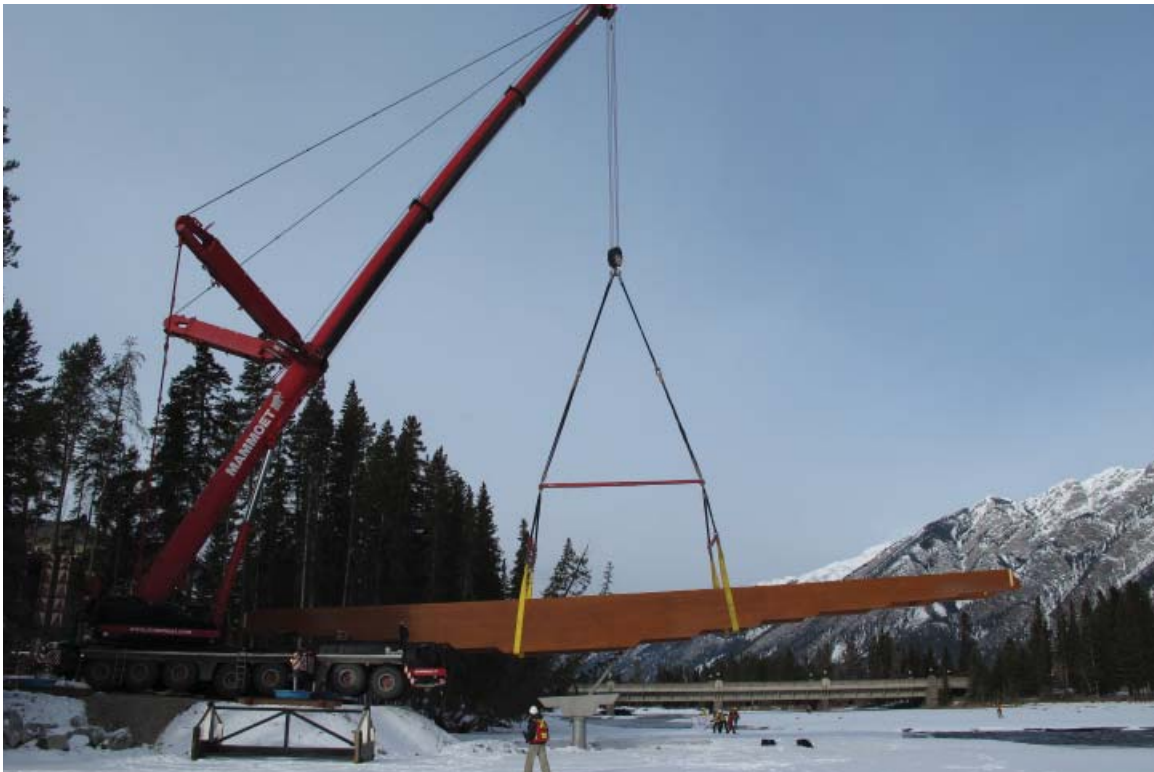
Figure 7: Installation of bridge end section. Photo Credit: StructureCraft Builders
