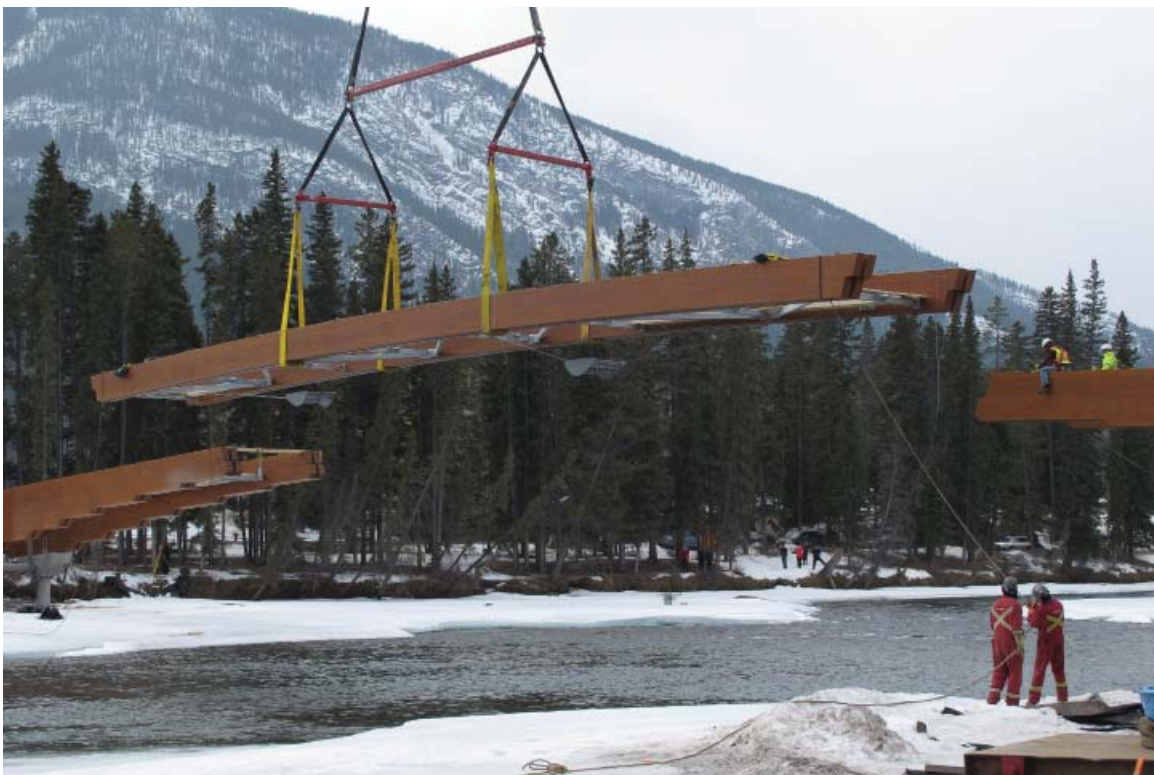
Figure 8: Installation of bridge center section. Photo Credit: StructureCraft Builders
