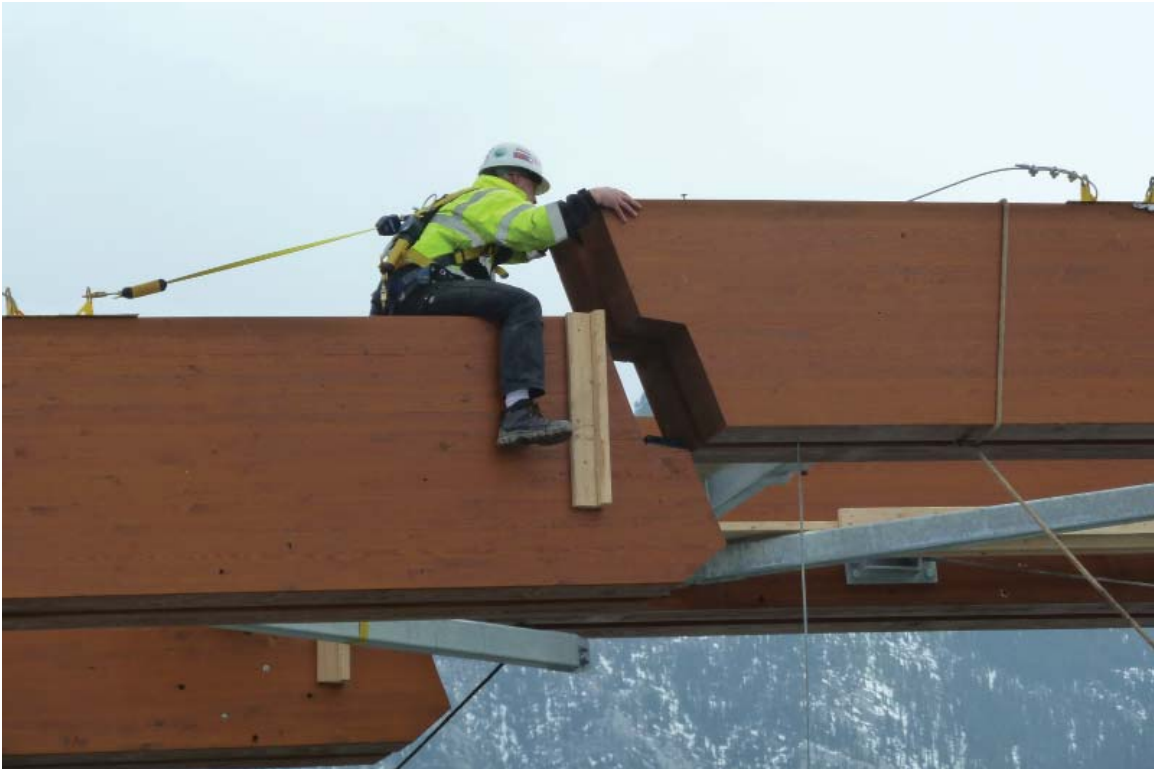
Figure 5: Fitting of bridge end and center sections. PhotoCredit: StructureCraft Builders
