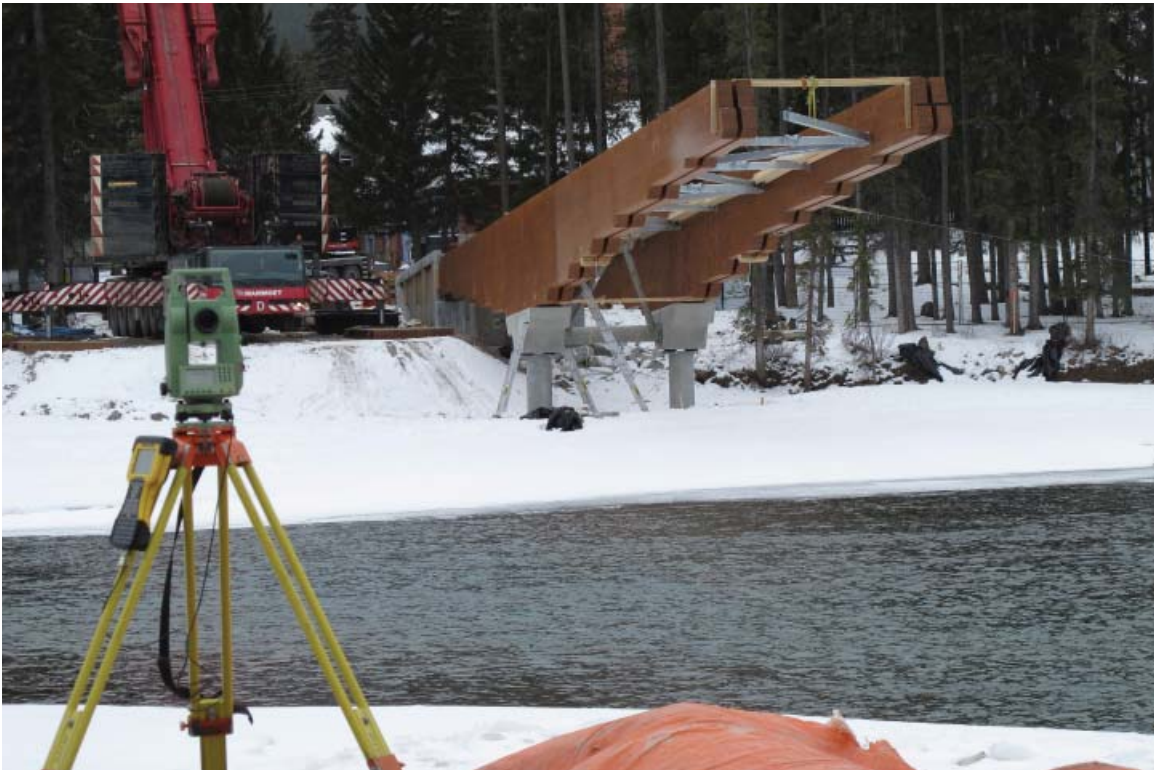
Figure 6: End section of bridge installed. Photo Credit: StructureCraft Builders
