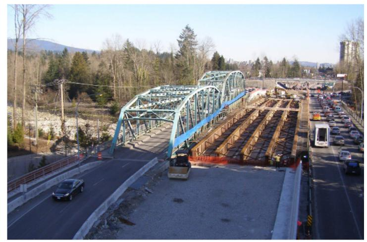
The **Move** The pre-built detour approaches were set to match the elevation of the bridge deck once it was set on sliders, so that once the bridge was in its new position, no vertical jacking was required; it was left on the sliding shoes for the life of the detour.
