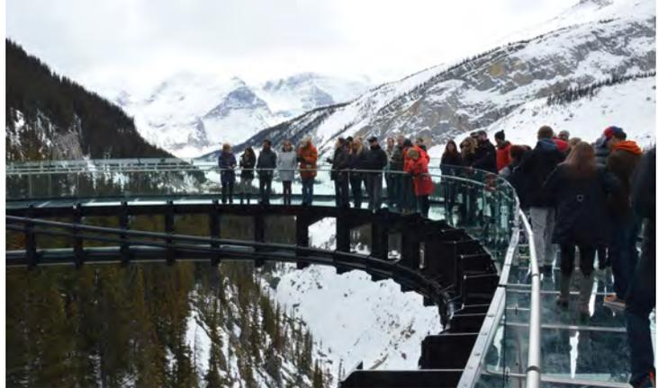
Like a diving board, the walkway structure is quite 'soft' so tuned mass dampers were utilized to mitigate vibration under dynamic loading to make it more comfortable for users. Wind deflectors were also added to the outer railings to ensure aerodynamic stability.
