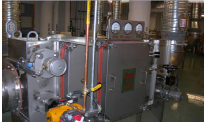
Figure 8: Next generation HEPA housing with integral bio seal dampers, and Autoscan technology
