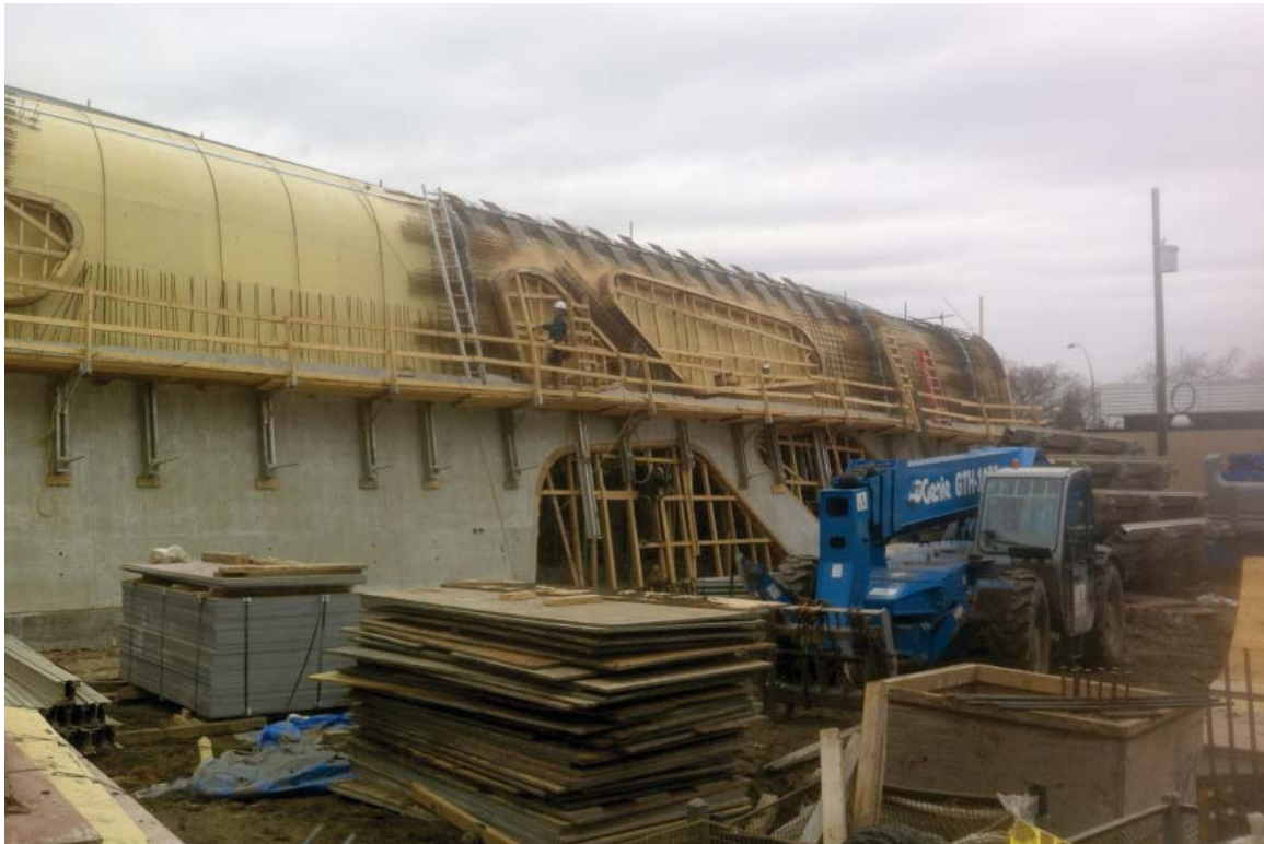
Figure 4: Construction of the exterior wall/ roof edge. Credit: Fast + Epp
