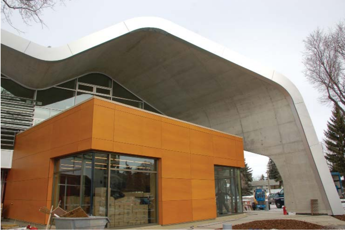
Figure 5: Large overhang using two-way stiffness of the concrete slab and geometric stiffness of wave form to provide support. Credit: Fast + Epp
