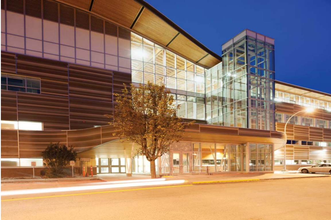
Figure 8: Exterior north entry. Photo Credit: Mathias Fast
