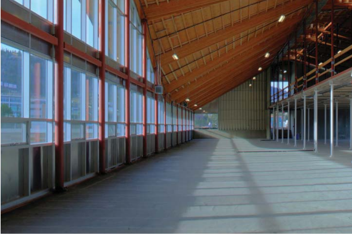
Figure 3: Completed shell prior to fit out. Photo Credit: Florian Maurer
