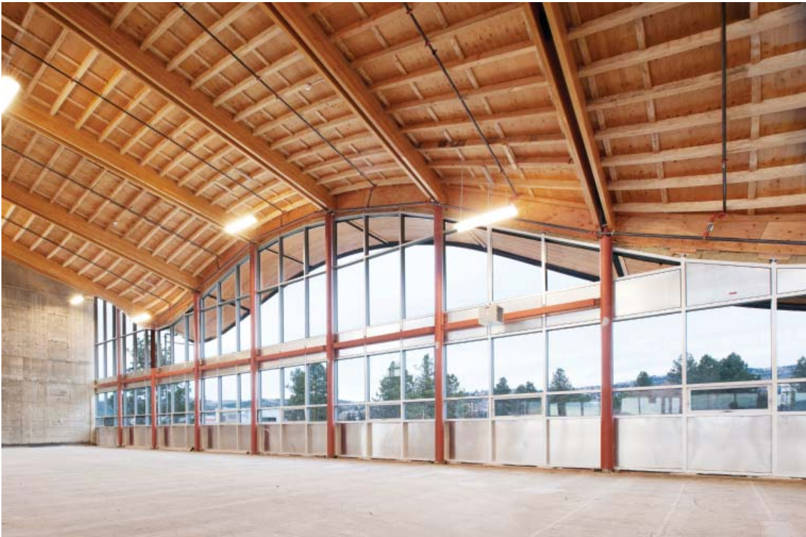
Figure 2: Installed panels prior to tenant improvements. Photo Credit: Mathias Fast
