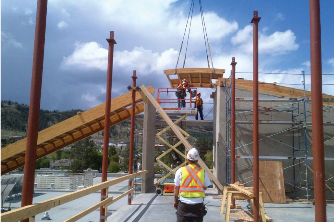
Figure 1: Pre-fabricated panel erection. Photo Credit: Yellowridge Construction
