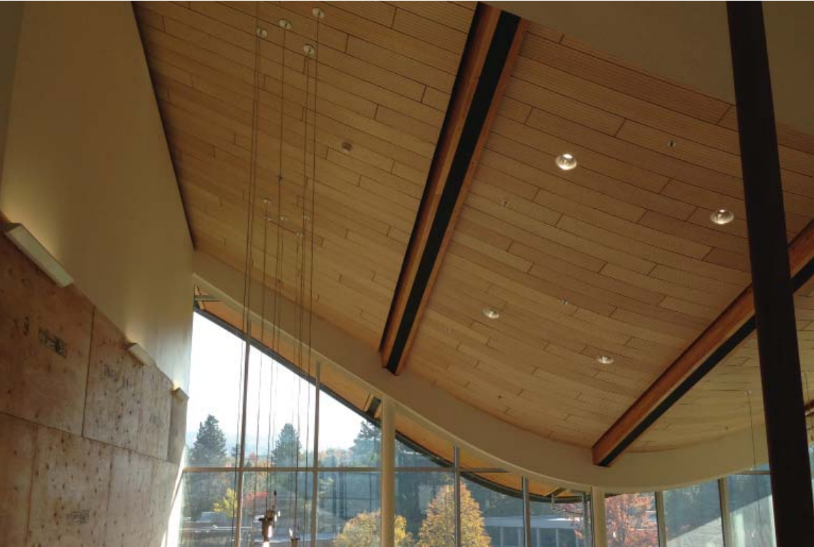
Figure 6: Interior lobby during fit out construction. Photo Credit: Mathias Fast
