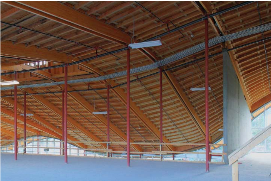
Figure 4: Completed shell prior to fit out. Photo Credit: Florian Maurer
