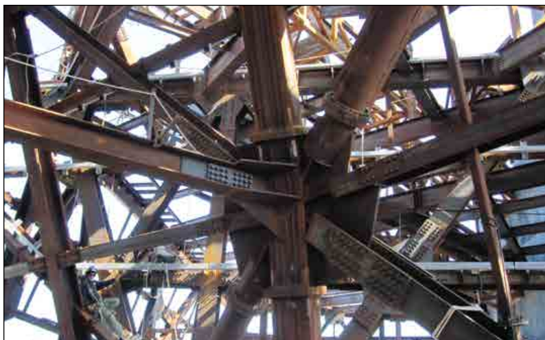
Shared super nodes with diagrid members between Mountain forms.
