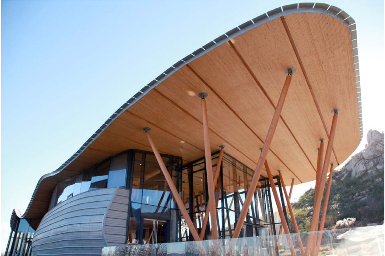
Figure 5: With 39 unique wood roof panels and 93 prefabricated columns, the Tsingtao Pearl Visitors Centre provides a warm user experience and welcome portal for the growing development in Qingdao, China. Photo Credit: Forestry Innovation Investment & Canada Wood
