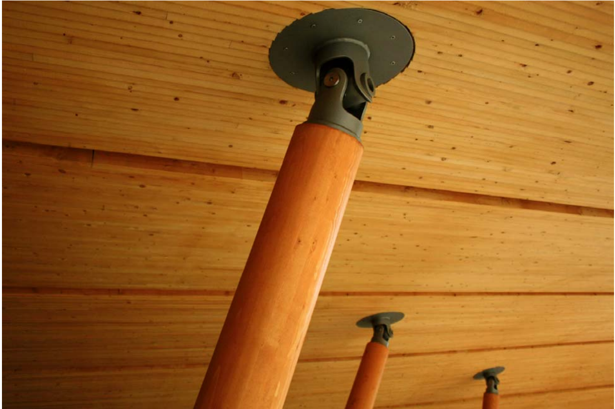
Figure 7: Intense design effort created a completely custom universal connector that would work for all 93 column orientations, at both the base and roof. Photo Credit: StructureCraft Builders
