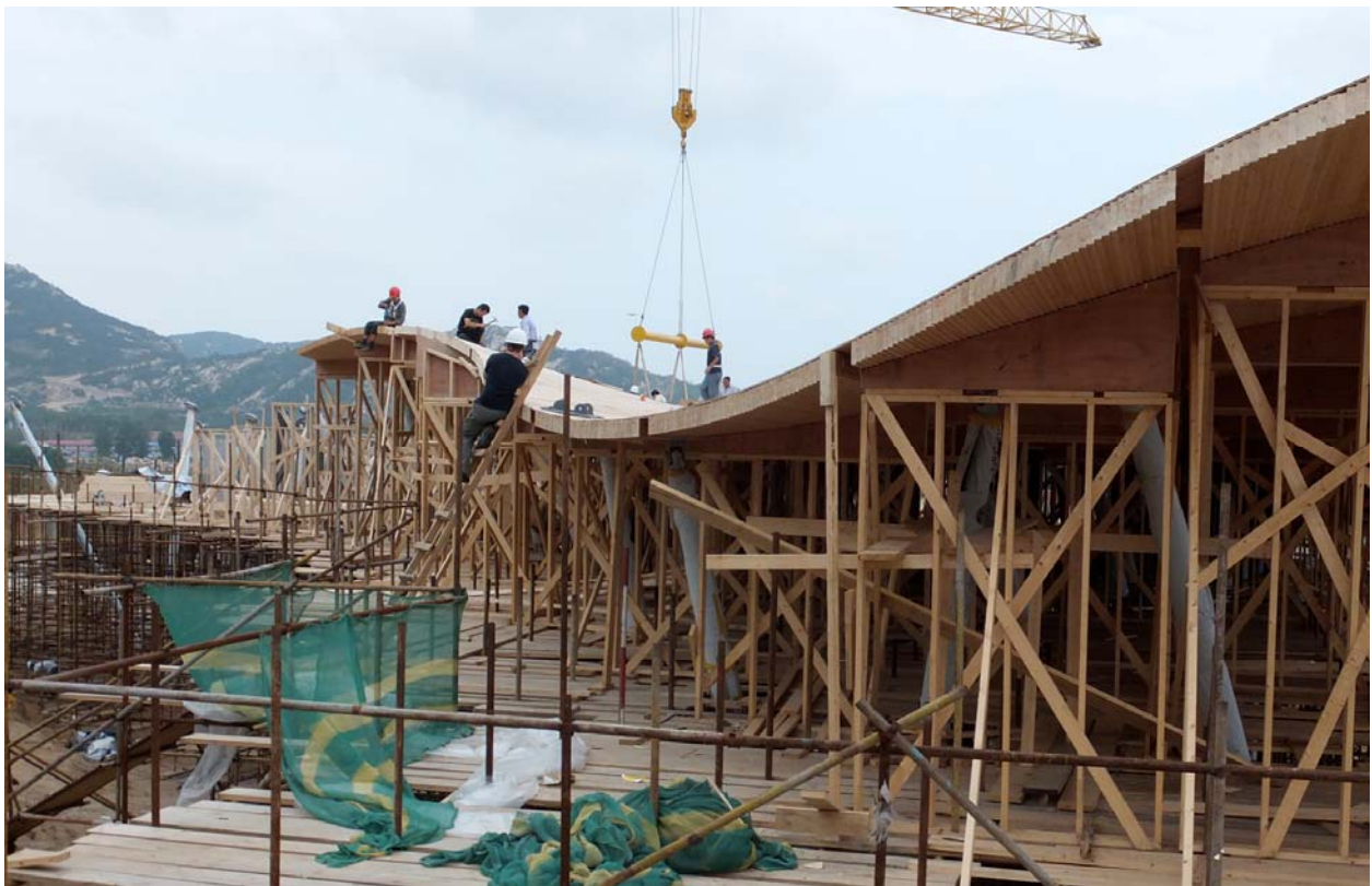
Figure 4: Construction crews rapidly erect the columns and roof panels on site, completing the building in adherence with the project’s tight schedule. The project was largely designed and constructed in eight months. Photo Credit: StructureCraft Builders
