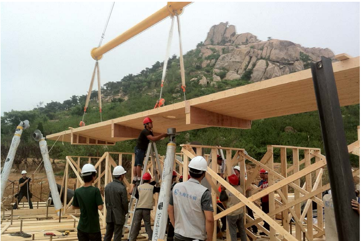
Figure 2: Crews erect the roof structure on site. Photo Credit: StructureCraft Builders
