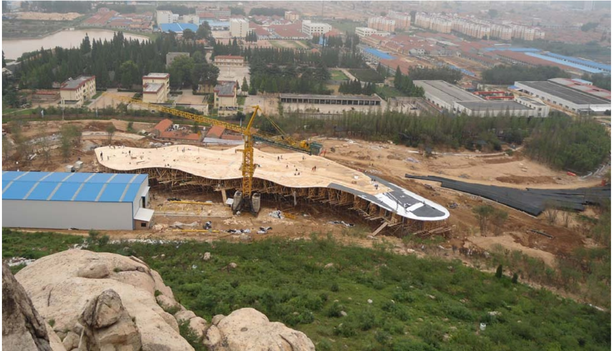
Figure 3: As the roof needed to have continuous strands of lumber for up to 40m, a scheme was developed to create visually “random” splicing, and panels were “stitched” together by loose pieces of lumber in place. Photo Credit: StructureCraft Builders
