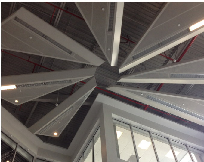
Ceiling mounted acoustic panels in entrance atrium.
