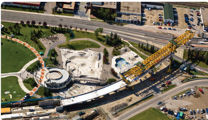
Elevated Guideway Construction
