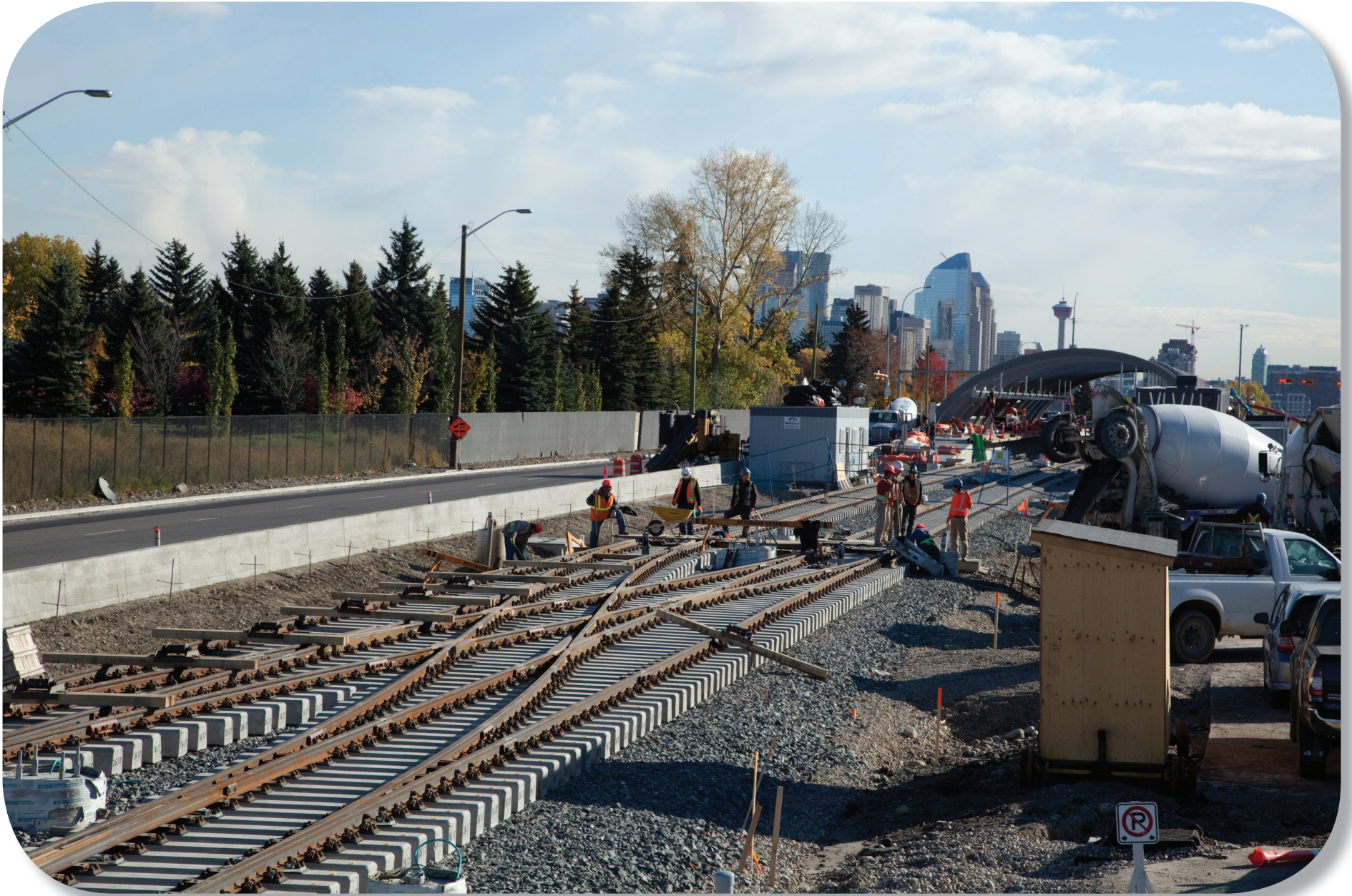
Construction of the Shaganappi Point Crossover
