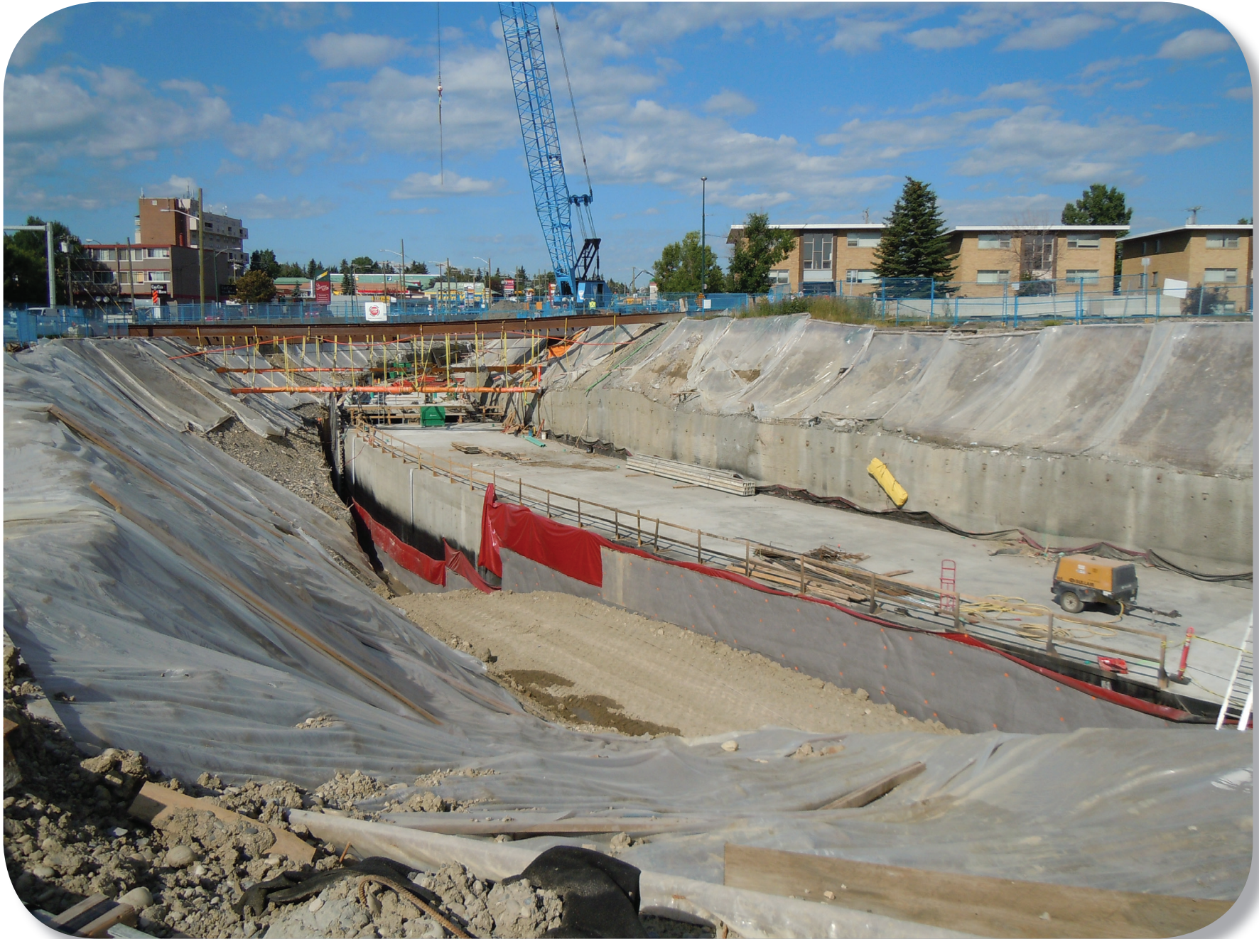
Cut and Cover Tunnel Construction
