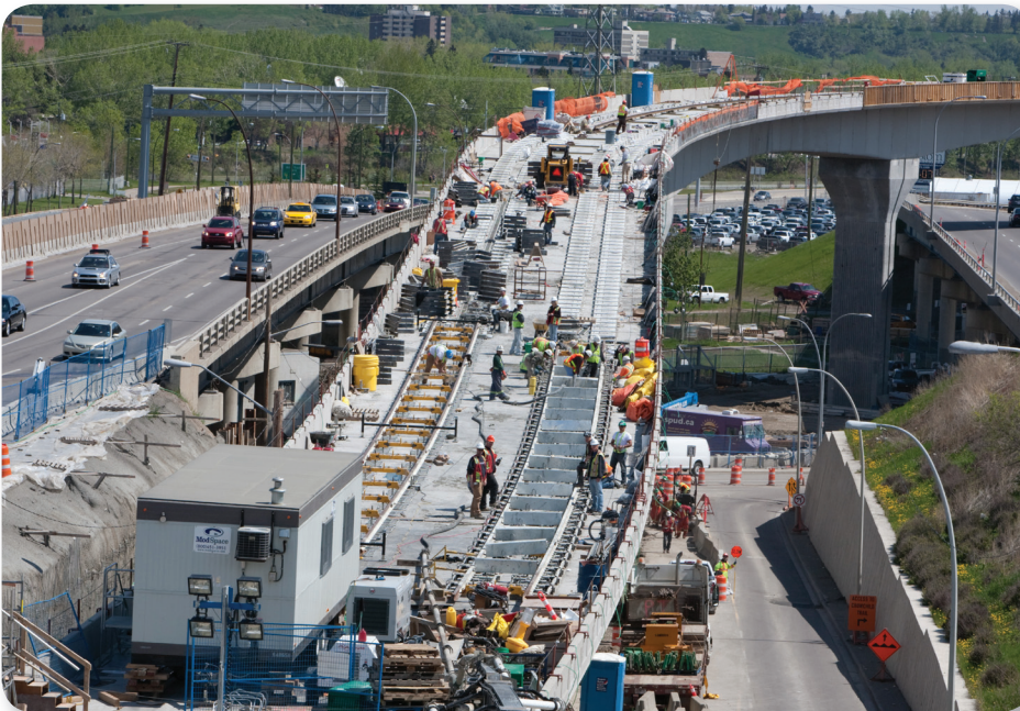
Direct Fixation Trackwork
