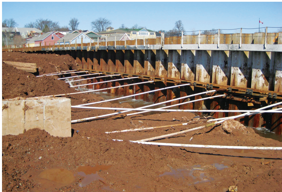
Charlottetown Convention Centre Site : Steel Sheet Pile and Seawall Tiebacks
