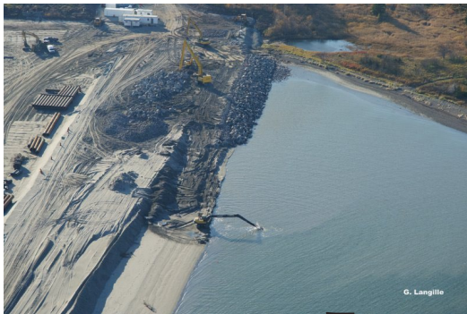
View of the revetment construction on the North Berm 5
