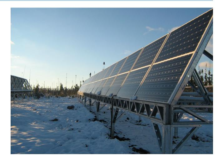
he use of solar electricity now reduces generator load and diesel use, providing significant environmental benefit.
