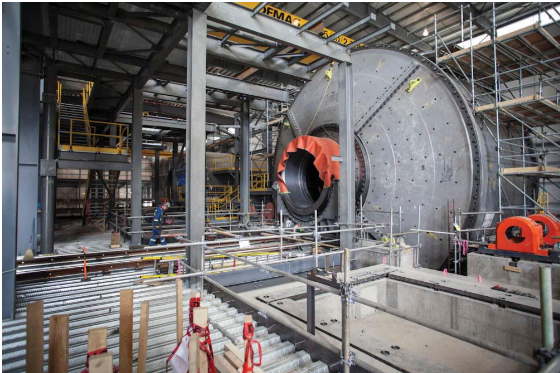
34" diameter SAG mill
