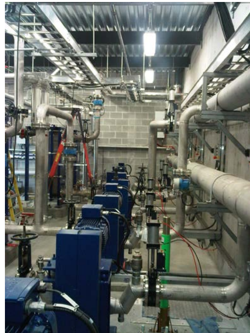
Figure 6 & 7 Views of Mechanical Room 2 showing the hot water recirculation pumps and heat exchangers (left) and the percolator recirculation pumps (right)
