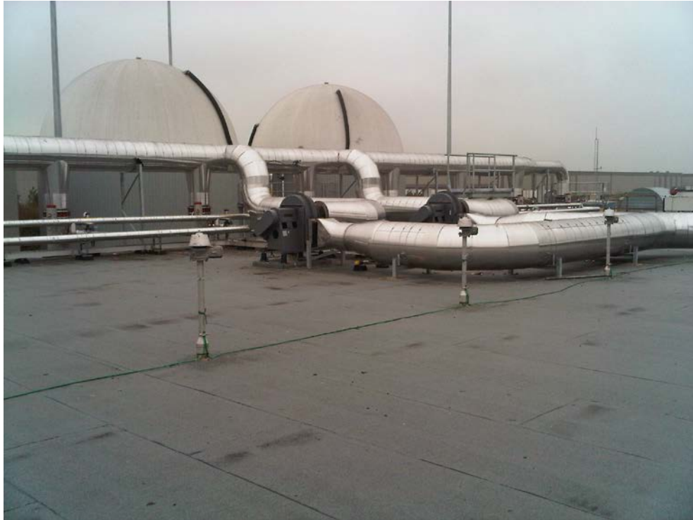
Figure 5 Top of the Percolators showing the Percolator Extraction Fans and Safety Vents (Methane Digesters in background)
